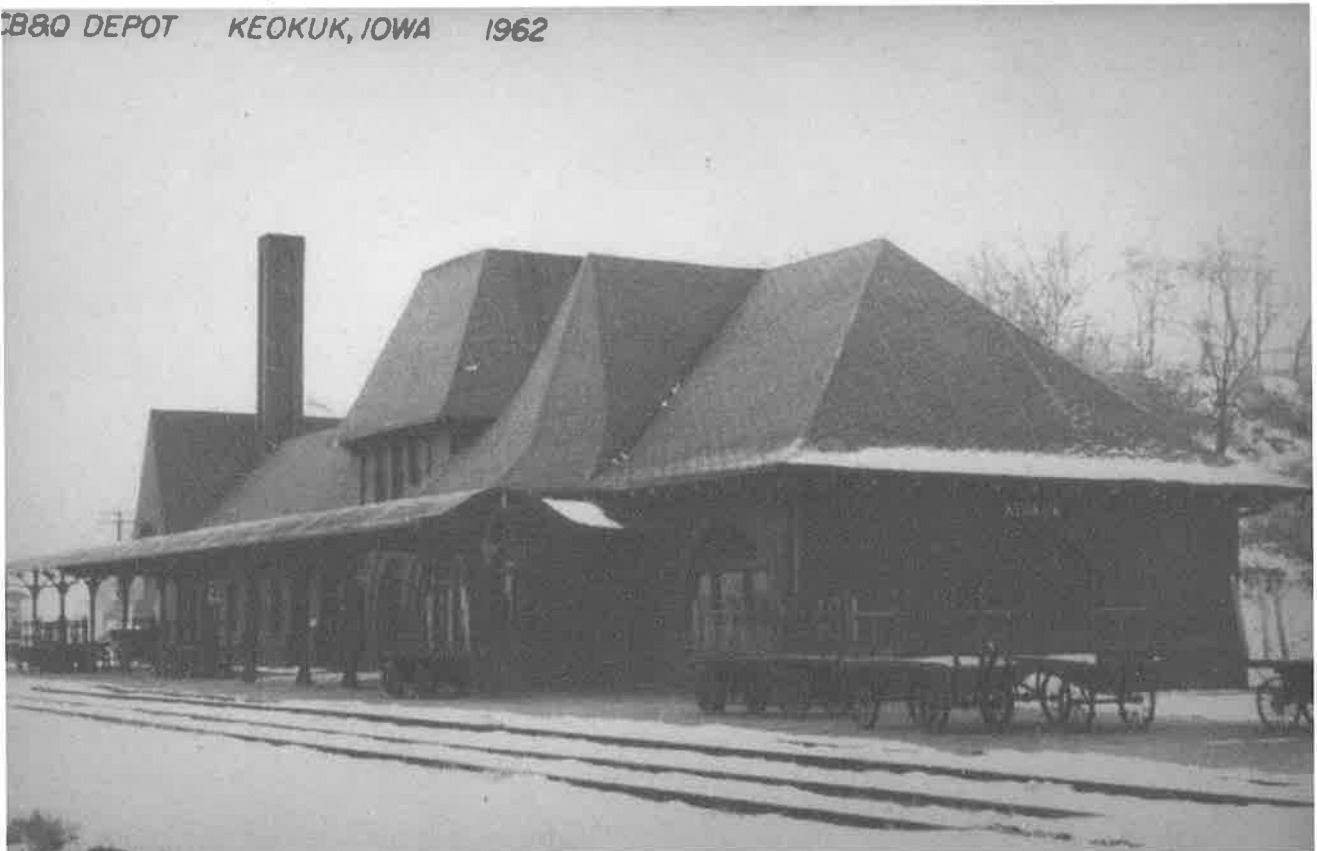
Figure 3: Looking at North and East façade of depot, 1962, Rob Adams Collection
