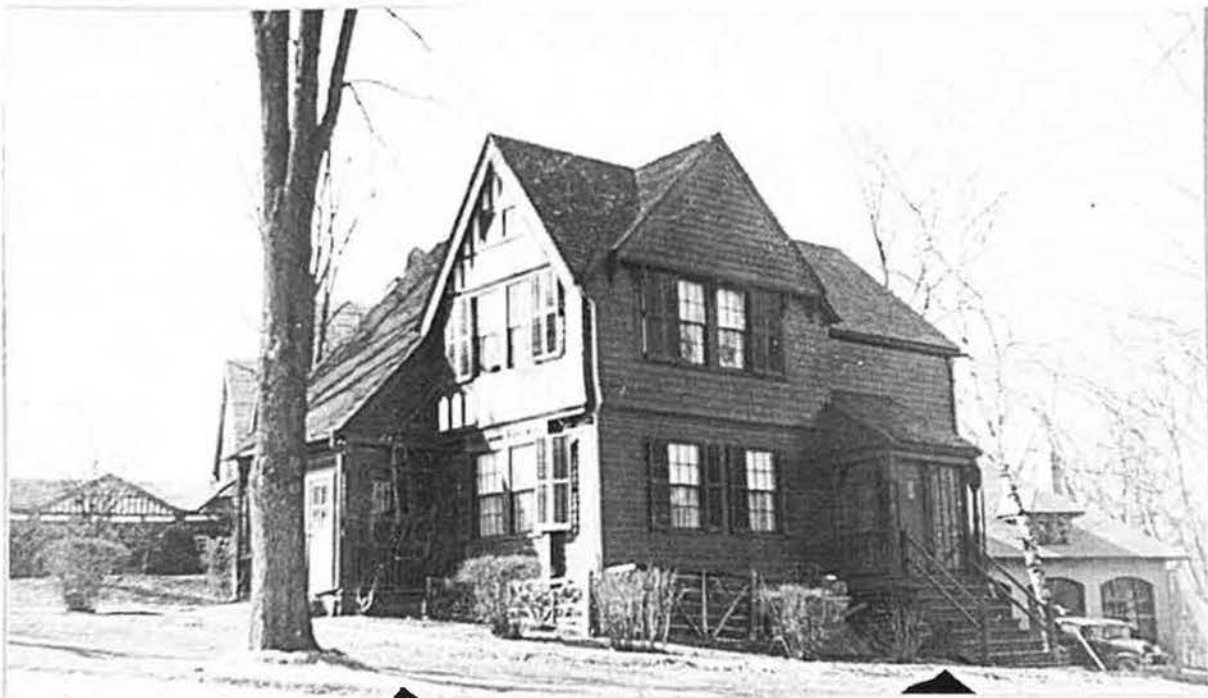
Figure 10. Caretaker's House, showing portion of Stable Carriage Shed and Garage/Workshop-Guest House, view southwest, 1938 (photo from Digital Commonwealth).
