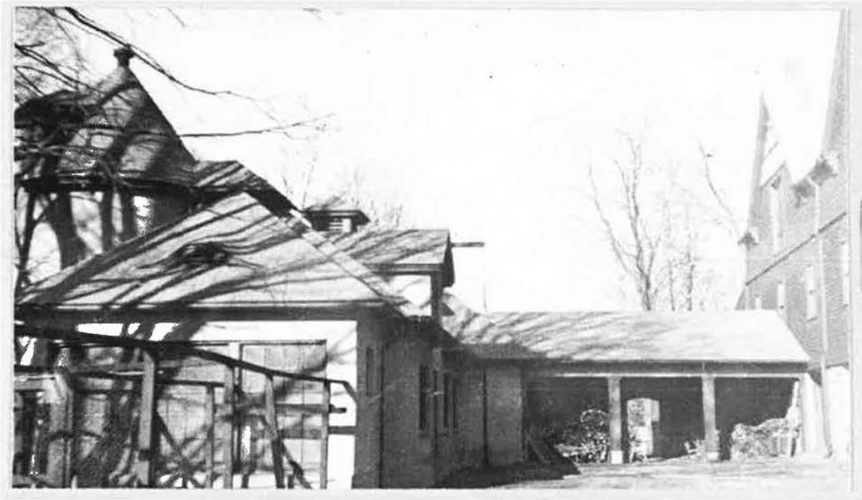
Figure 9. Garage/Workshop-Guest House and Stable, view north, 1938 (photo from Digital Commonwealth).
