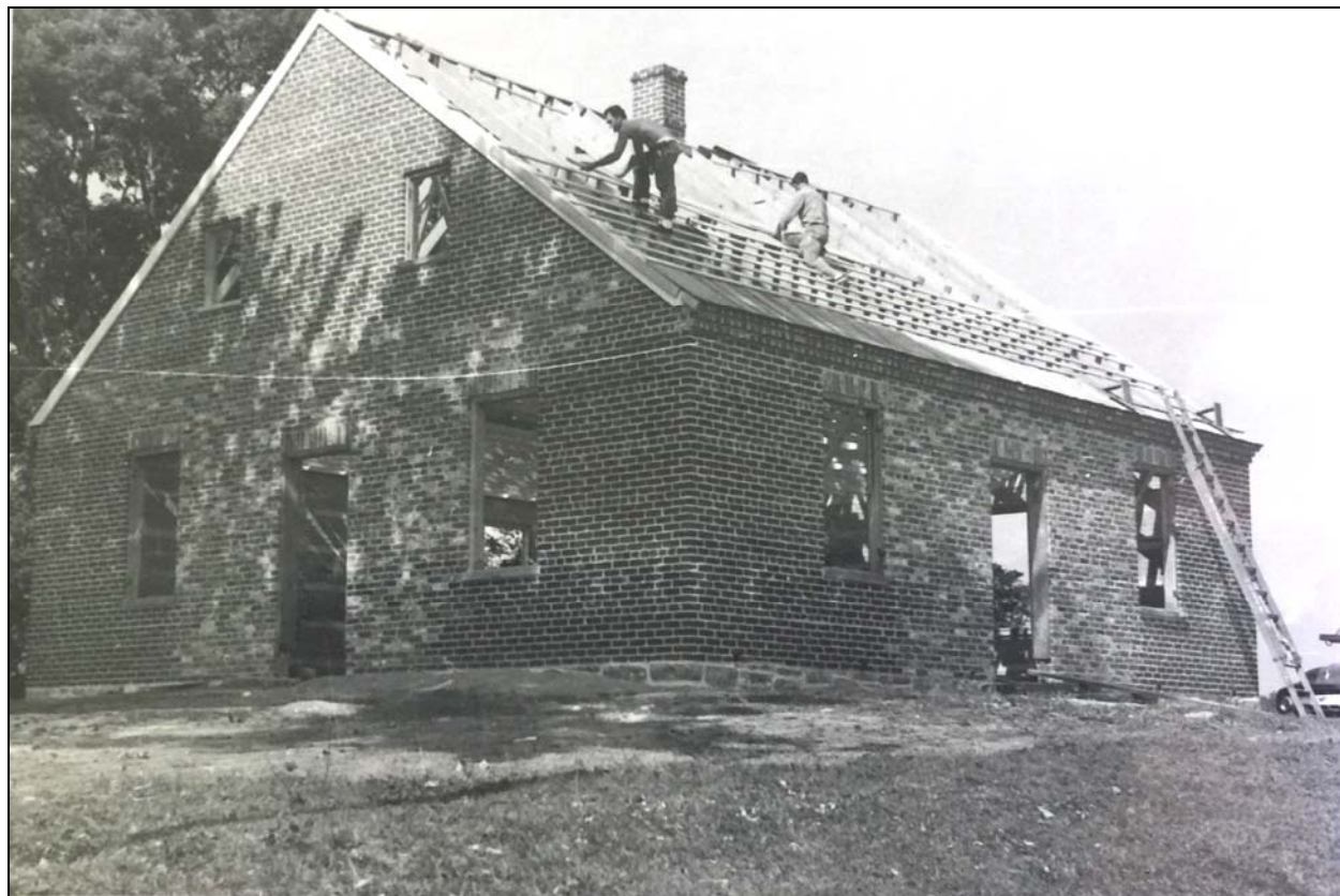
Figure 6. The Dunker Church during reconstruction, 1961. Source: Antietam National Battlefield Archive.
