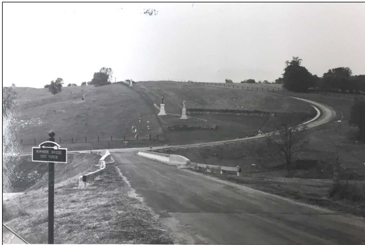
Figure 25. Rodman Avenue Bridge and realigned Branch Avenue, 1966. Source: Antietam National Battlefield Archives
