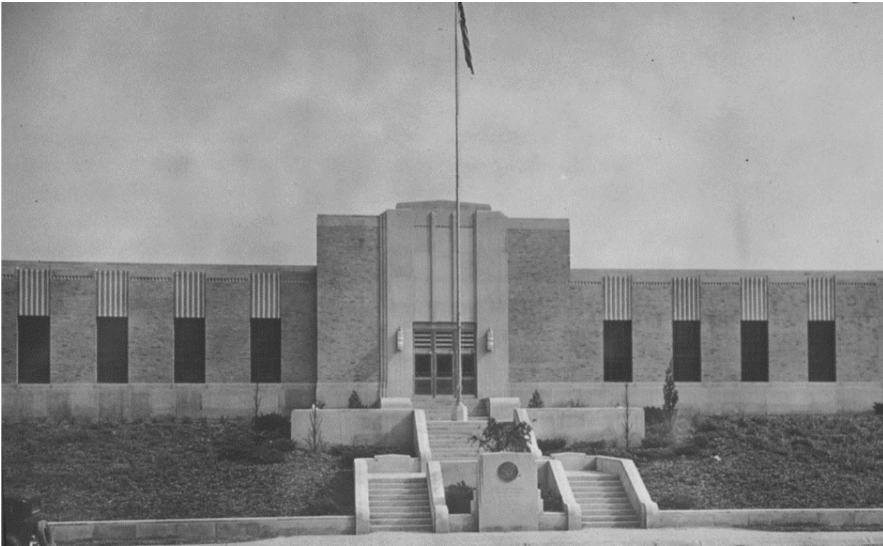
1938 Burns & McDonnell Water Treatment Plant, Cincinnati, Ohio. This plan established much of the vocabulary observed on Seaholm. 25
