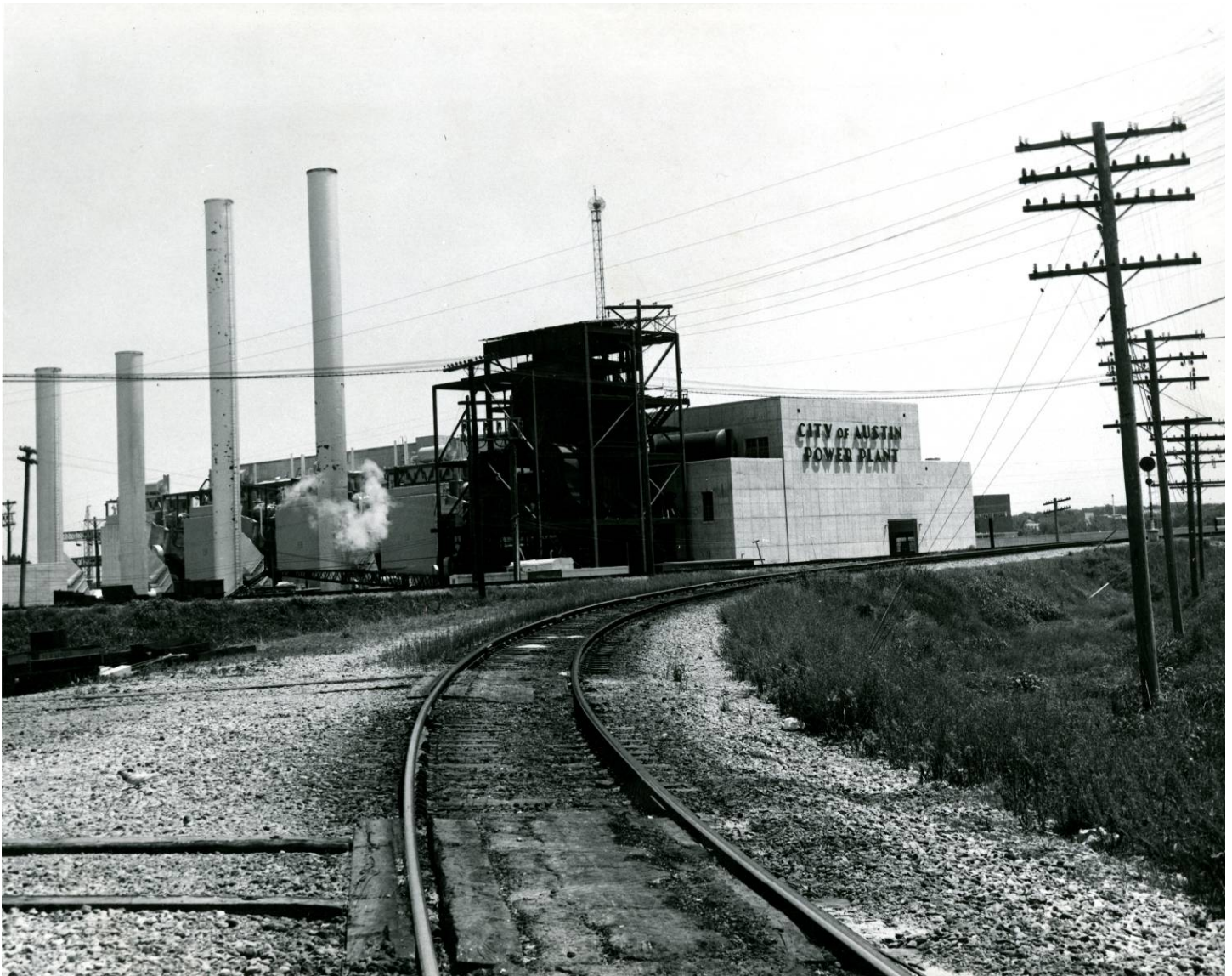
Seaholm Power Plant, 1955.
