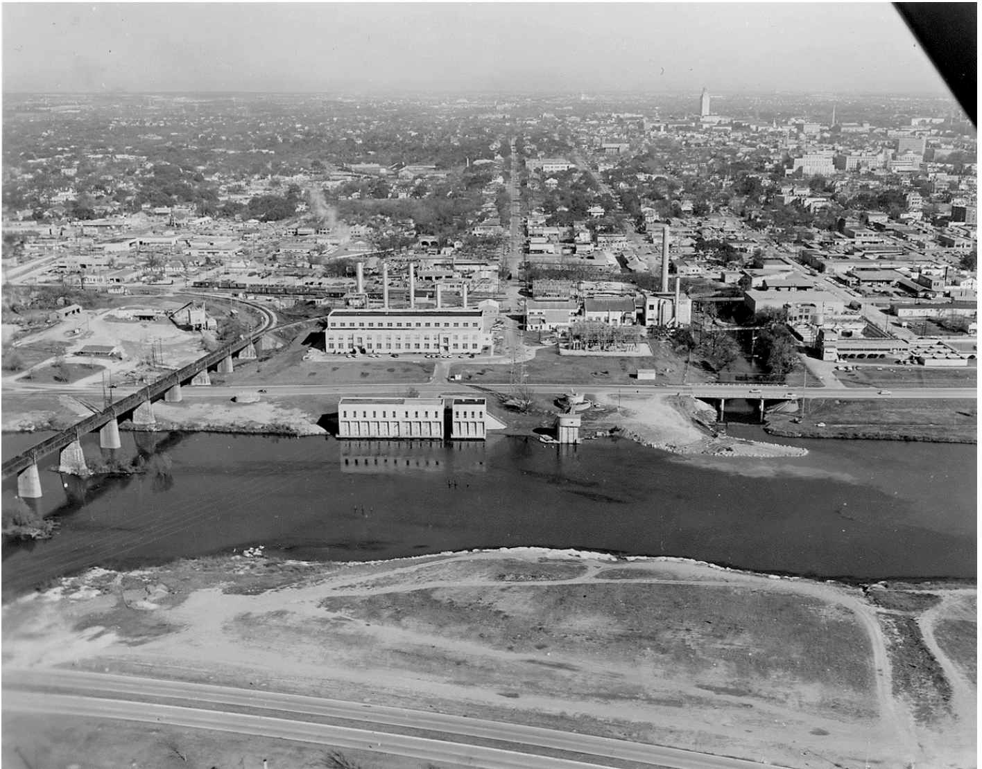
1984 Aerial photograph of south façades of Turbine Generator Building and Water Intake Building, and Earthen Island, camera facing north
