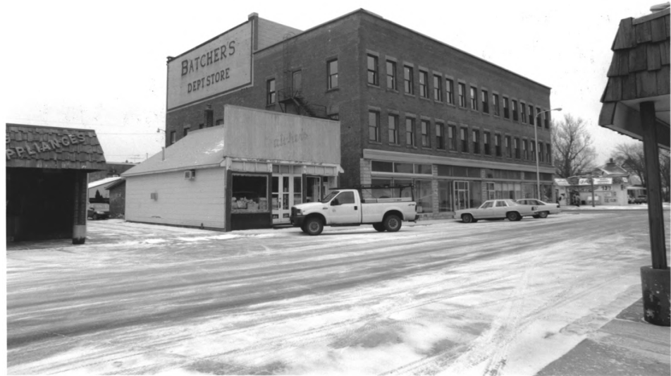
Batcher Opera House Block Todd Co., Mn 014752-23/23A
