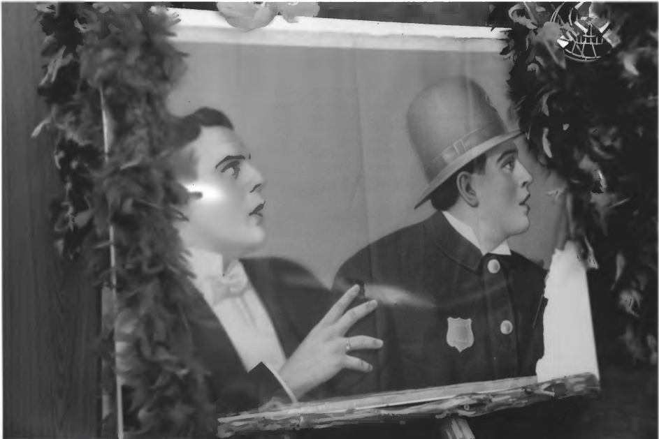
Batcher opera House Block Todd Co., Mn 014753-21A/22
