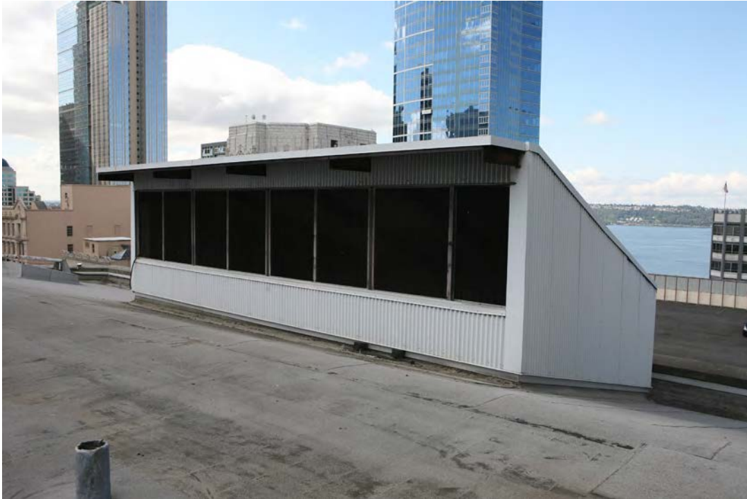
23 of 27. Bon Marche Building, roof, looking west.
