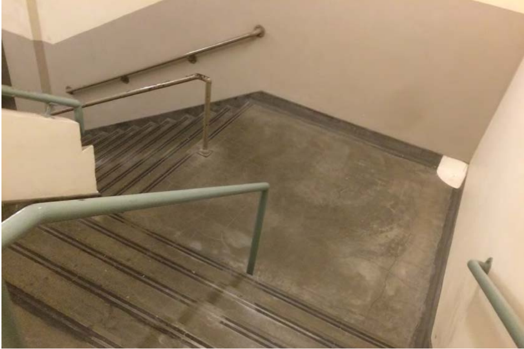
27 of 27. Bon Marche Building, stairwell example.
