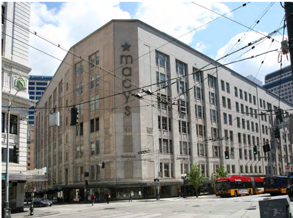
6 of 27. Bon Marche Building, looking southeast at Third Avenue (west) and Olive Way (north) elevations.
