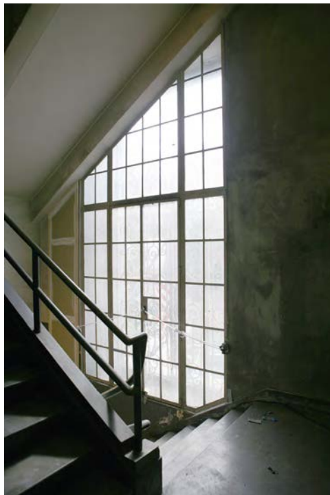
26 of 27. Bon Marche Building, stairwell, southern portion.
