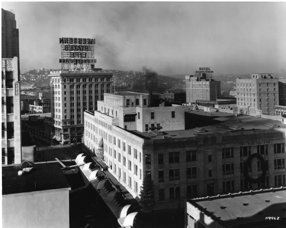
Historic Photograph 8. Ca. 1930s. View of the rooftop and elevator penthouse of the Bon Marche Building, looking northeast. Source: Museum of History and Industry.
