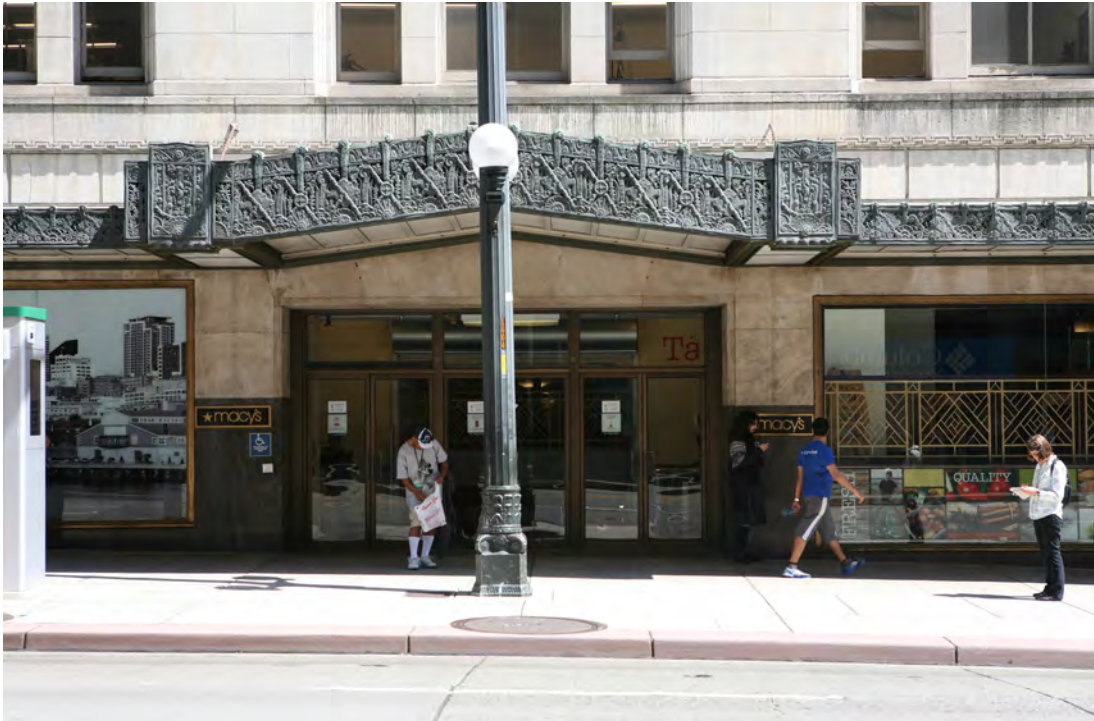
7 of 27. Bon Marche Building, central Third Avenue (west elevation) entrance.
