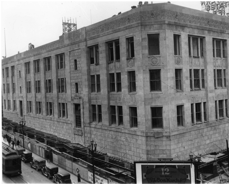
Historic Photograph 5. 1929. Bon Marche Building under construction (near completion). Source: Museum of History and Industry.
