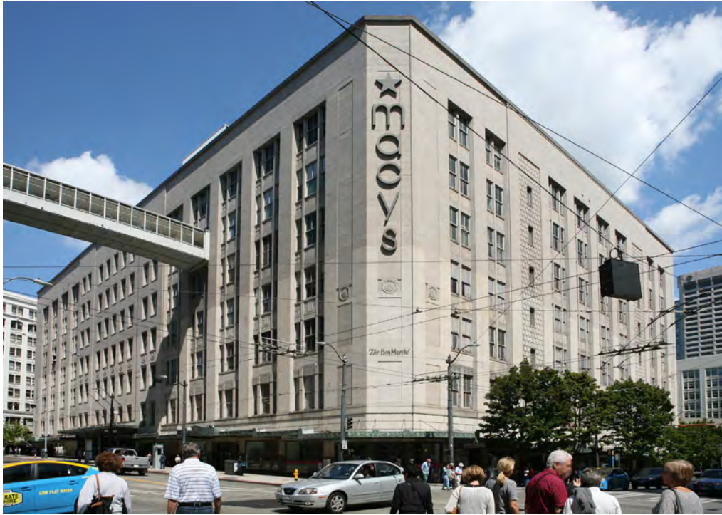
5 of 27. Bon Marche Building, looking northeast at Pine Street (south) and Third Avenue (west) elevations. Note the sky-bridge connecting to the building, constructed 1960.
