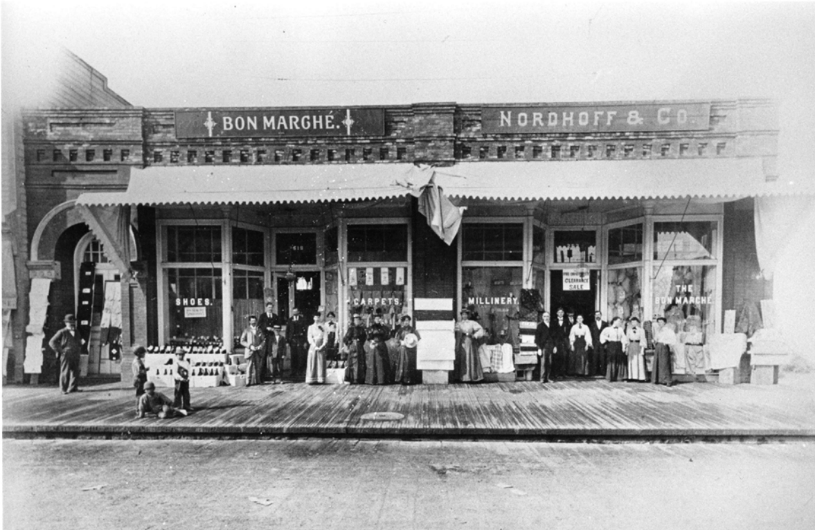
Historic Photograph 1. Ca. 1890s. First Bon Marche store located on Front Street (now First Avenue) and Cedar Street in Seattle's Bell Town neighborhood. Source: University of Washington Special Collections.
