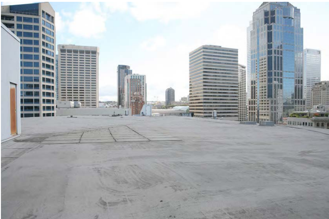
24 of 27. Bon Marche Building, roof, looking east.
