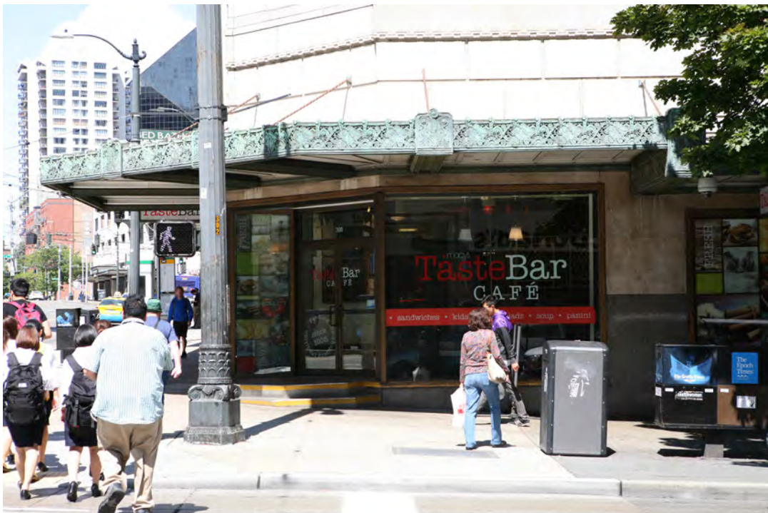
4 of 27. Bon Marche Building, southwest corner (Third Avenue and Pine Street) entrance with intact marquee.
