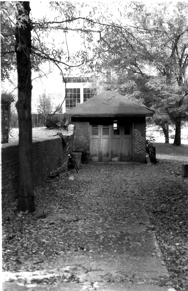
#6 of 10 McConnell, Chancellor T.M.'s House Chattanooga, Hamilton Co TN
