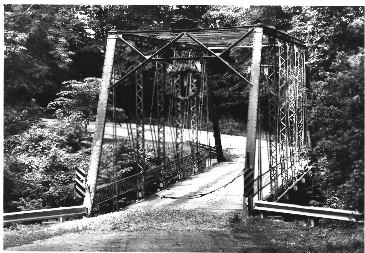
WILSON BRIDGE, CARROLL COUNTY, INDIANA - 2
