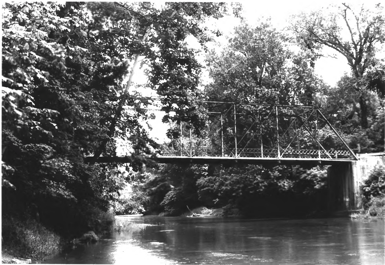
WILSON BRIDGE, CARROLL COUNTY, INDIANA - 4
