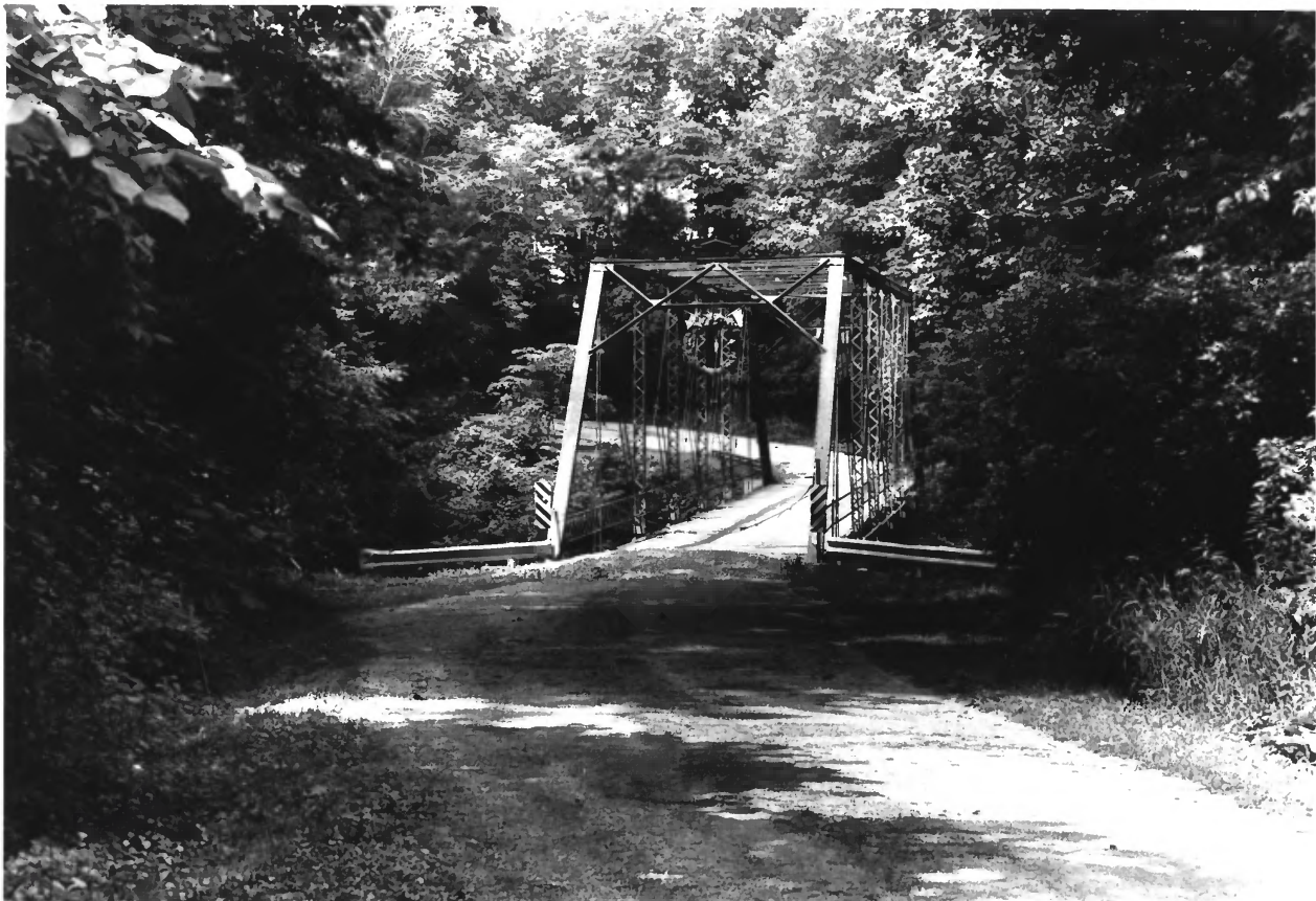
WILSON BRIDGE, CARROLL COUNTY, INDIANA - 3
