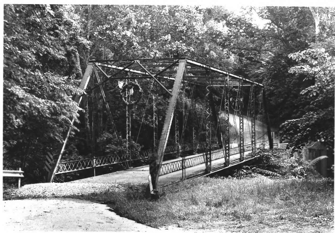
WILSON BRIDGE, CARROLL COUNTY, INDIANA - 1
