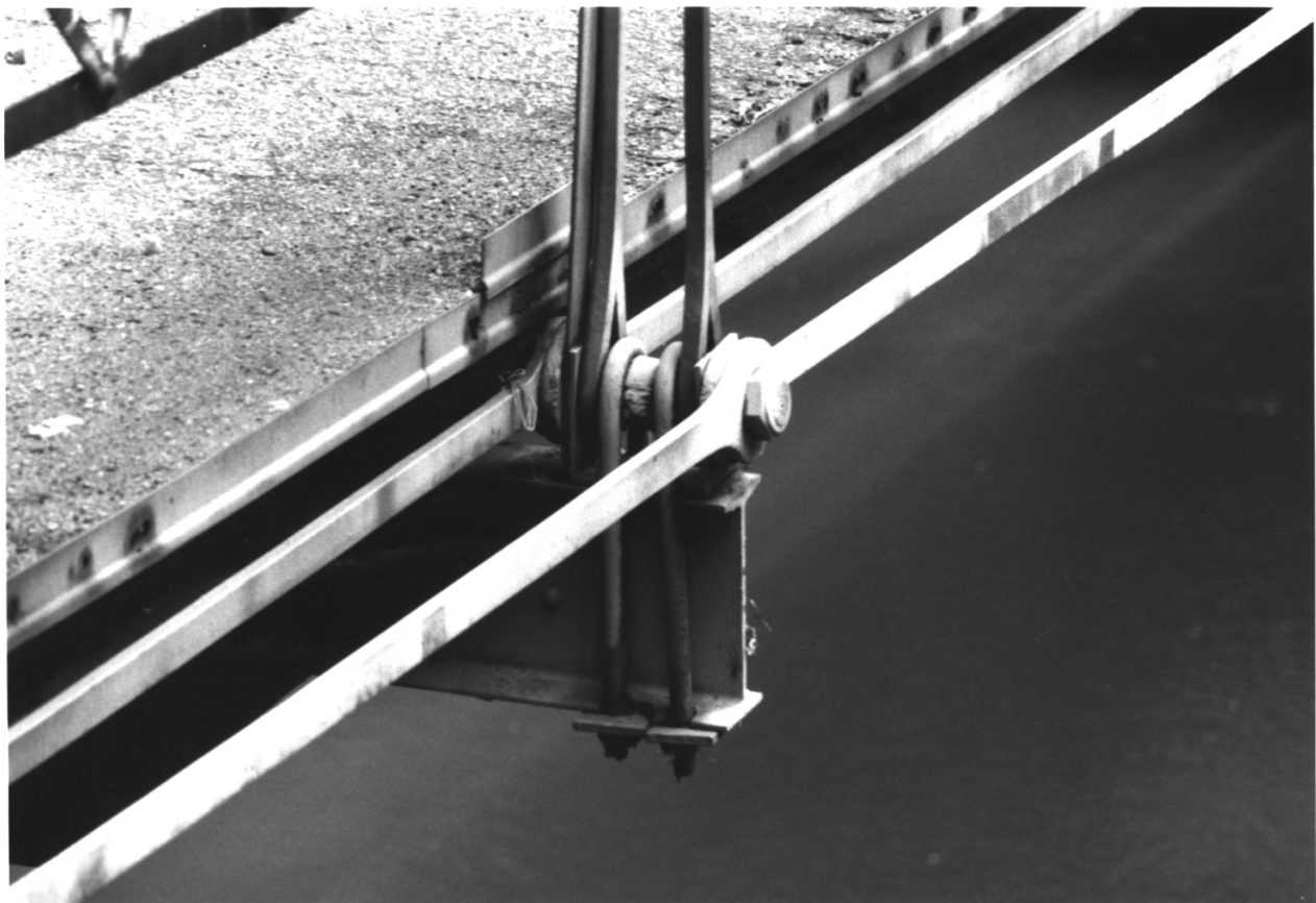
WILSON BRIDGE, CARROLL COUNTY, INDIANA - 6
