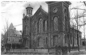
Photograph 1. Late 18 th /early 19 th C. Note three entranceways in ground floor of the principal façade and domed cupola on smaller tower. Parsonage (1889) to the left. Photographer unknown. Image courtesy of the Madison Historical Society.
