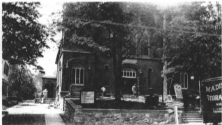
Photograph 2, 1924. Renovations underway. Notice that the tower entranceways are being replaced with windows. Photograph taken by Mrs. Huldah I. Peck. Courtesy of the Madison Historical Society.
