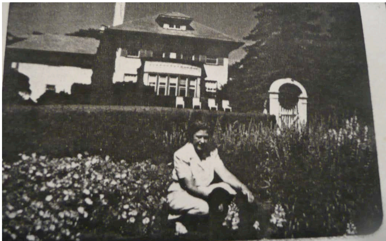
Figure 1 Historic Photo, south façade, view to north
