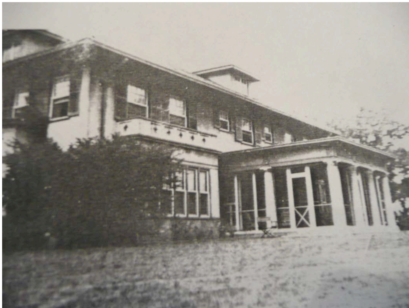
Figure 2 Historic Photo, east façade, view to west
