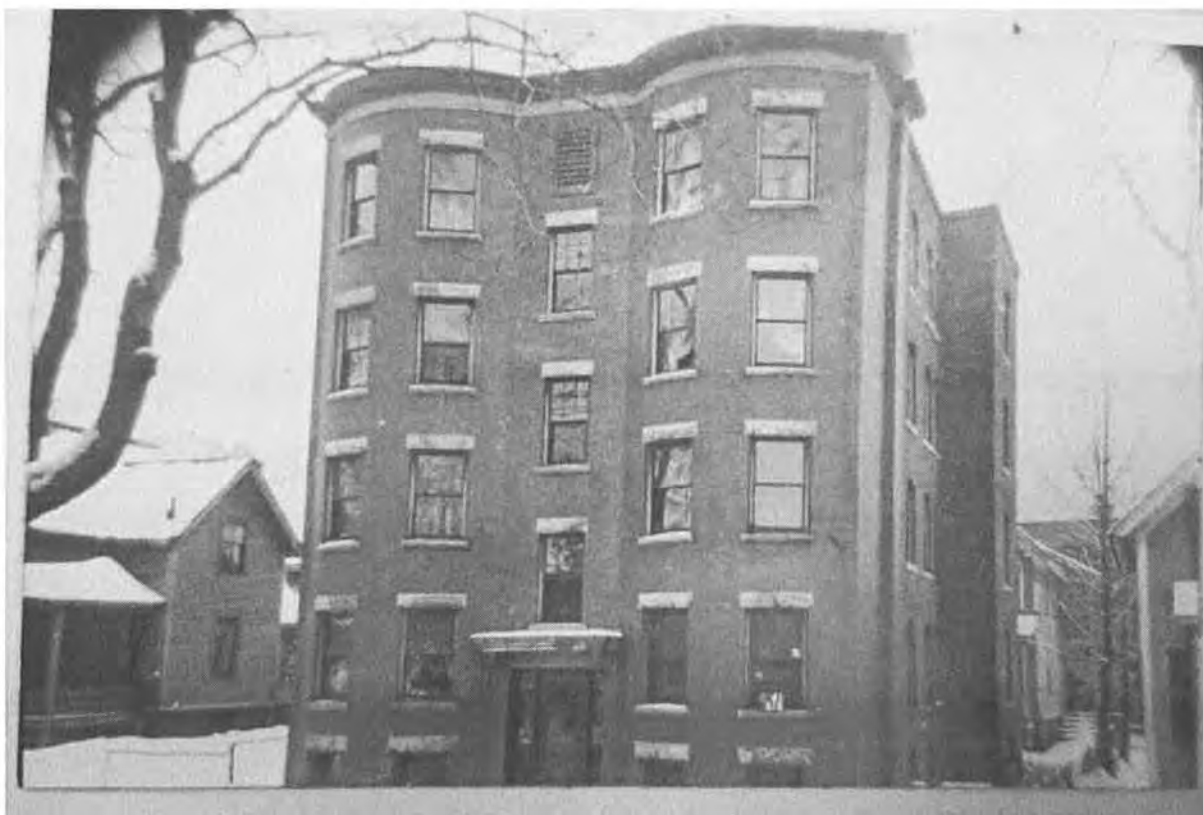
Figure 7. 1939 photograph (north elevation) of Adams Apartment Building, courtesy Springfield Building Department.
