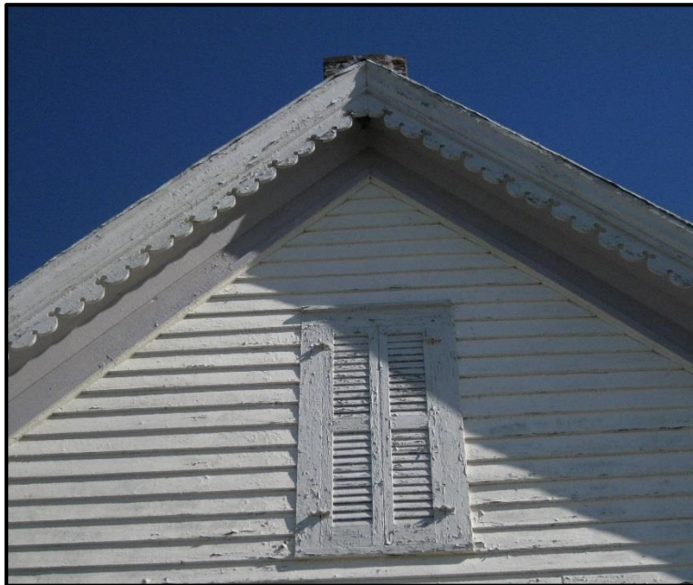
Figure 3. Detail of roof trim, west gable
