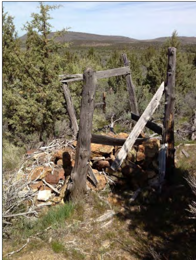
Photo 22 of 26: Detail of fence jack at east side of Barn Orchard, view north (2 May 2014).
