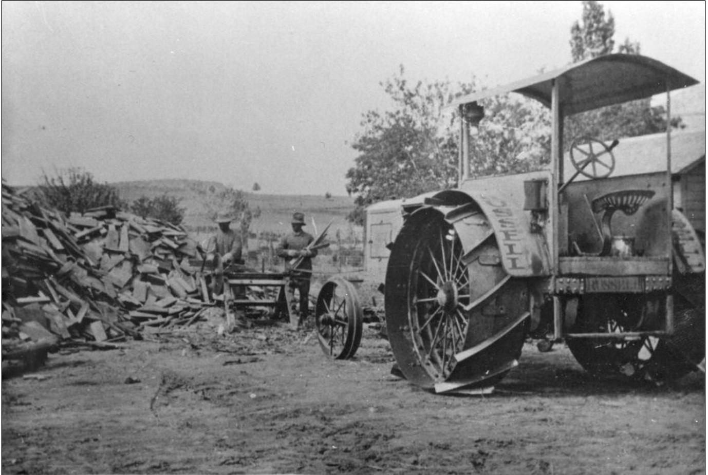
Figure 14 of 16: Cyrus family members cutting shakes to length using a Russell Big Boss 20-40 tractor for power and a belt driven buck saw, circa 1920.
