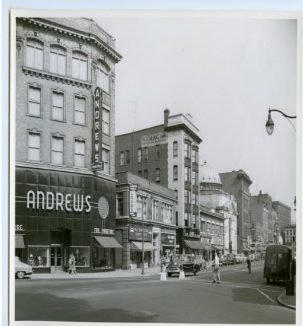
15. Main Street. New Britain, Hartford County, Connecticut. Southwest view, Photo taken in the 1960s, Photo courtesy of the New Britain Local History Room.
