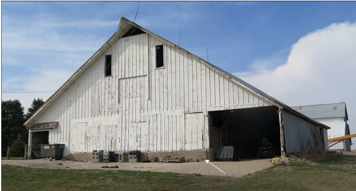
Figure 10. The south face of the late 19 th -century Middle Barn looking NNW. It is called the show barn because it was used to provide cattle shows for prospective buyers who would visit from around the state and country. Show days at the Pleasant View Farm were festive events. The original stone foundation is visible through the concrete on this side of the barn (white arrow).
