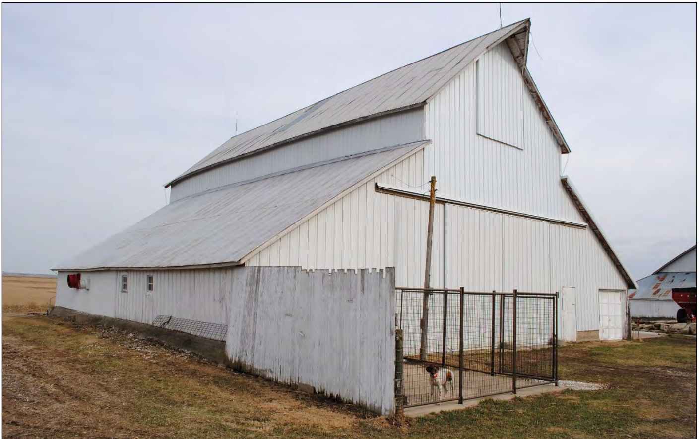
Figure 32. Monitor roof barn looking ESE at the façade and north side of the barn. Photograph taken by Tallgrass Archaeology LLC, 04/12/2018.
