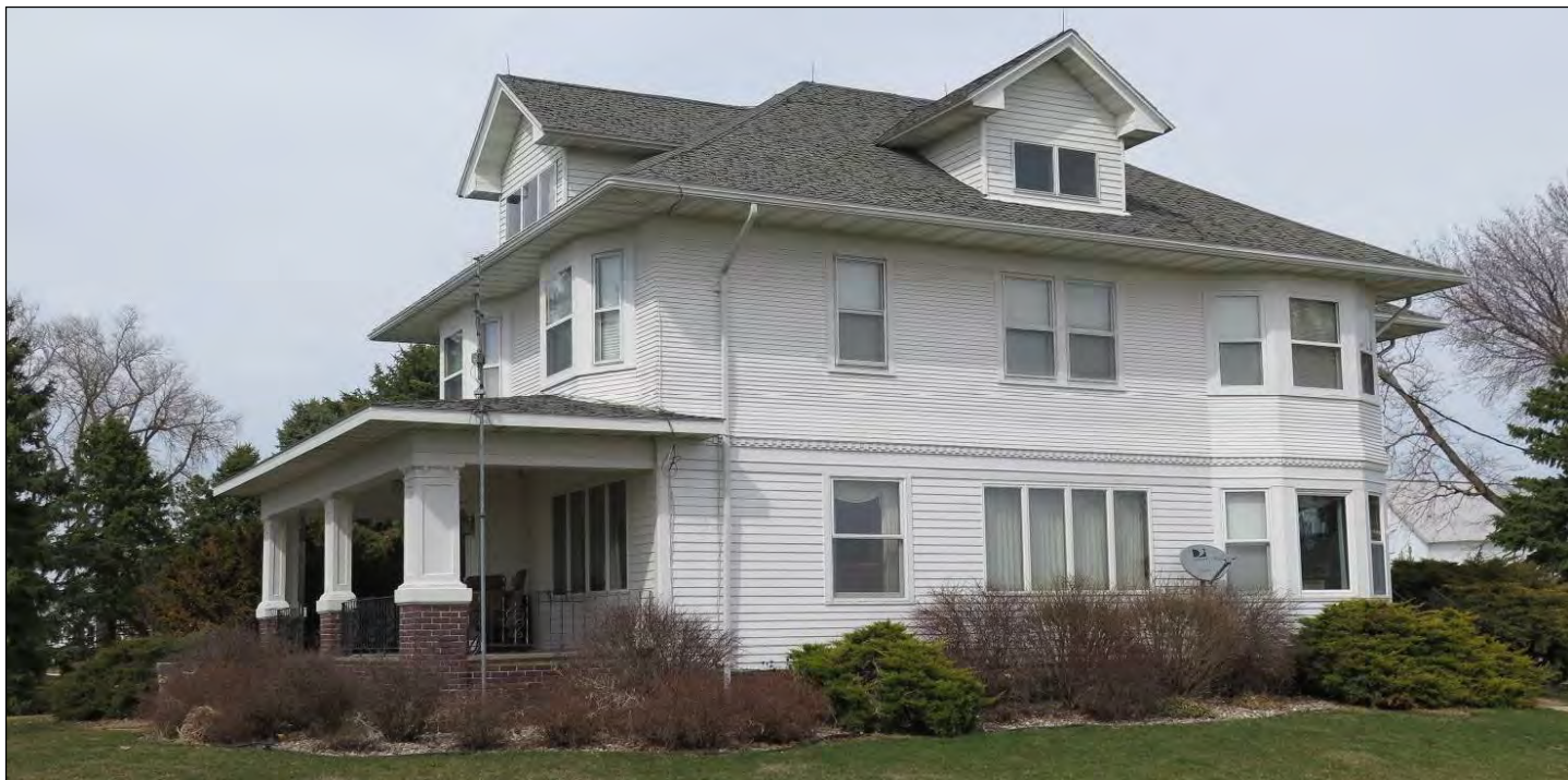
Figure 3. 1913 farm house looking NNE. Notice the west-facing front porch with brick detailing, west- and south-facing dormers, the two-story rounded bay window on the south side and the two single-story rounded bay windows above the front porch; and the denticulated board separating the first and second stories on the exterior of the house. Photograph taken by Tallgrass Archaeology LLC, 04/12/2018.
