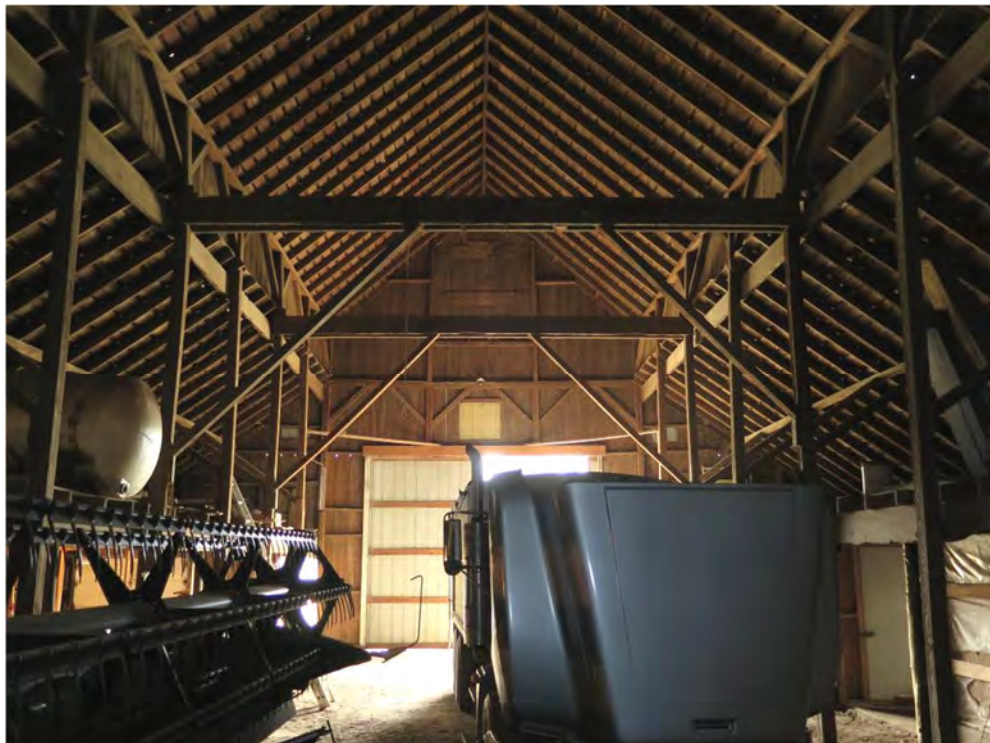
Figure 37. Interior of North Barn looking west in the center aisle and showing the two full interior bents. Photograph taken by Tallgrass Archaeology LLC, 04/13/2018.
