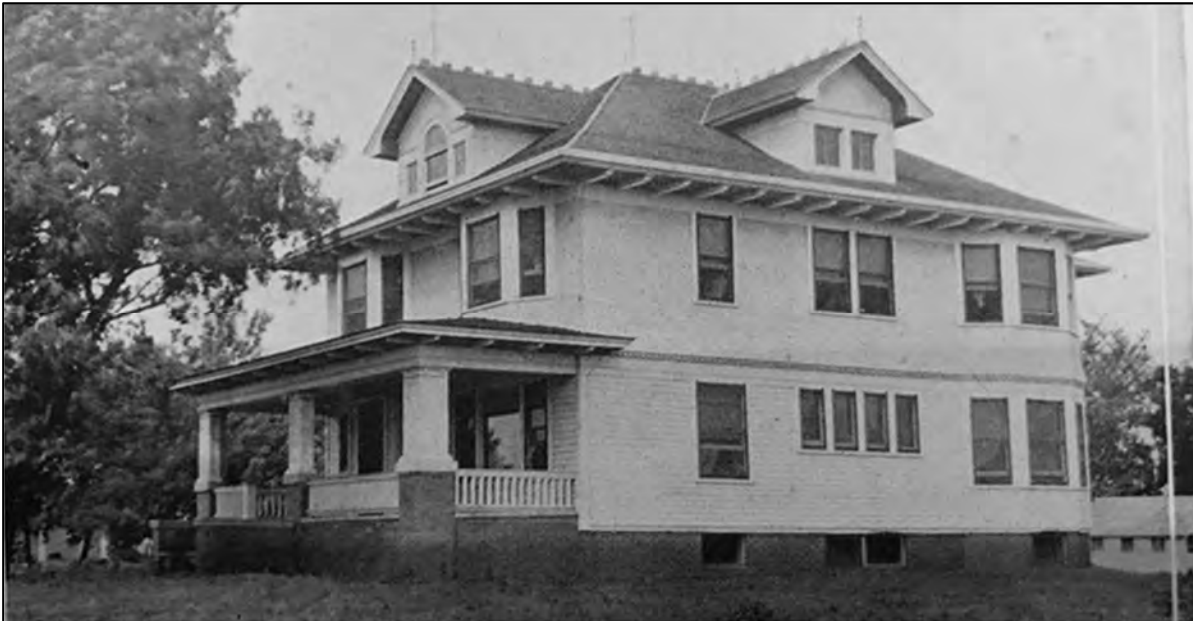
Figure 65. Historic photograph of the Ryan house at Pleasant View Farm. Note the Palladian window in the front dormer, the original windows on the front porch and on the south side center, the roof ridge cresting, and the wooden railing on the front porch, now replaced or removed. The corbels under the eaves so visible in this photograph are still in place but not as highly visible in the current photograph in Figure 66 because of the gutters. Copy of photograph provided by Abbie Ryan Nelson.
