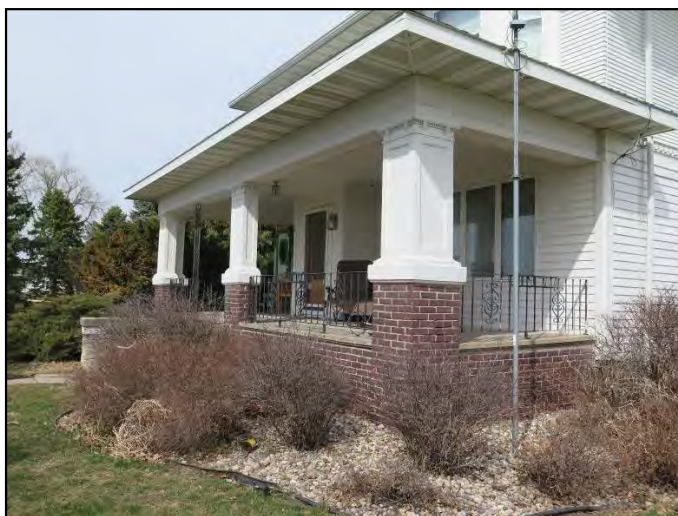
Figure 5. Front porch of 1913 house looking NNE.
