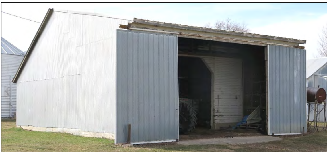
Figure 41. Machine Shed looking WNW and showing the older frame machine shed on the interior of the outer metal shed shell. Photograph taken by Tallgrass Archaeology, 04/12/2018.
