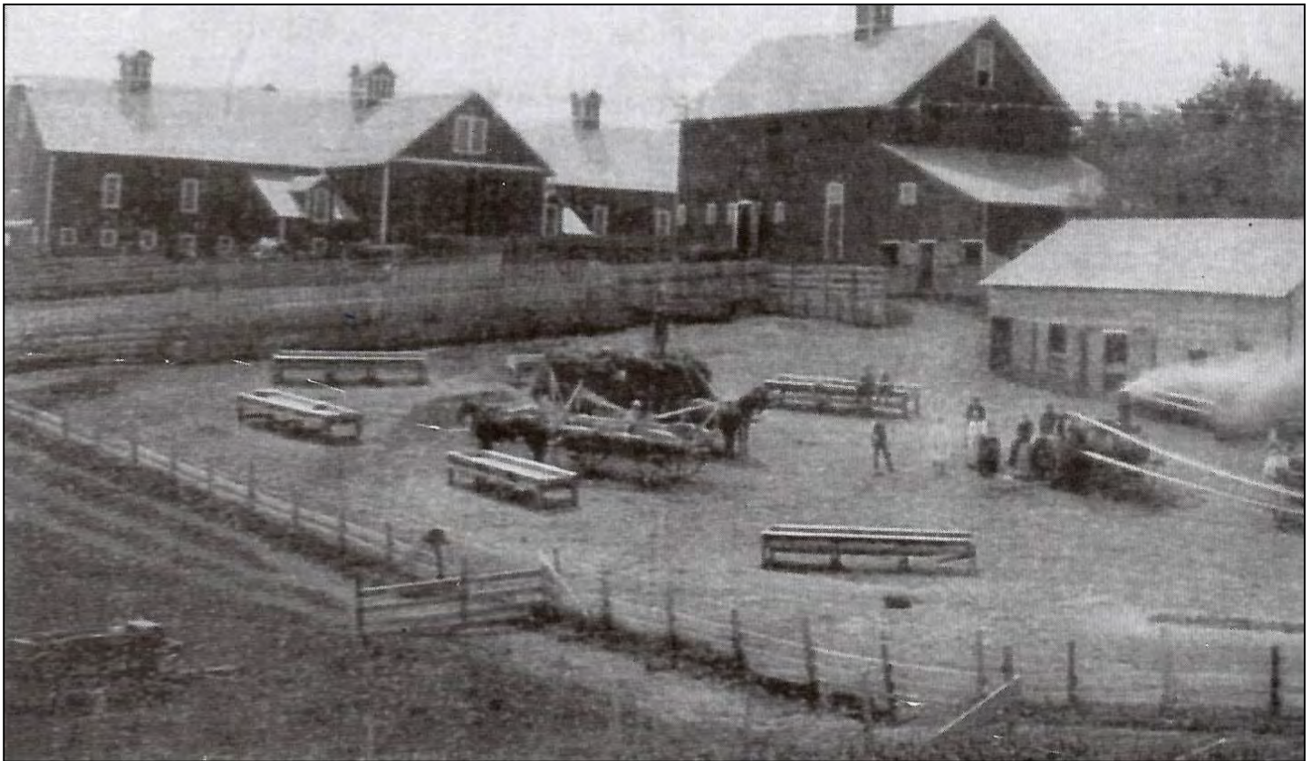
Figure 61. This 1898 photograph of the barns on the Long Branch Farm shows the cross-shaped barn (upper left) and a gabled transverse frame barn (upper right) that may have inspired the T-shaped barn construction on Pleasant View Farm. The cross-shaped barn had become a T-shaped barn by the late 20th century and burned down circa 2010. The above view was taken from the north looking southwest. What is now 2200th Street in Shelby County is the lane that extends between the two barns. Source: American Angus Hall of Fame.
