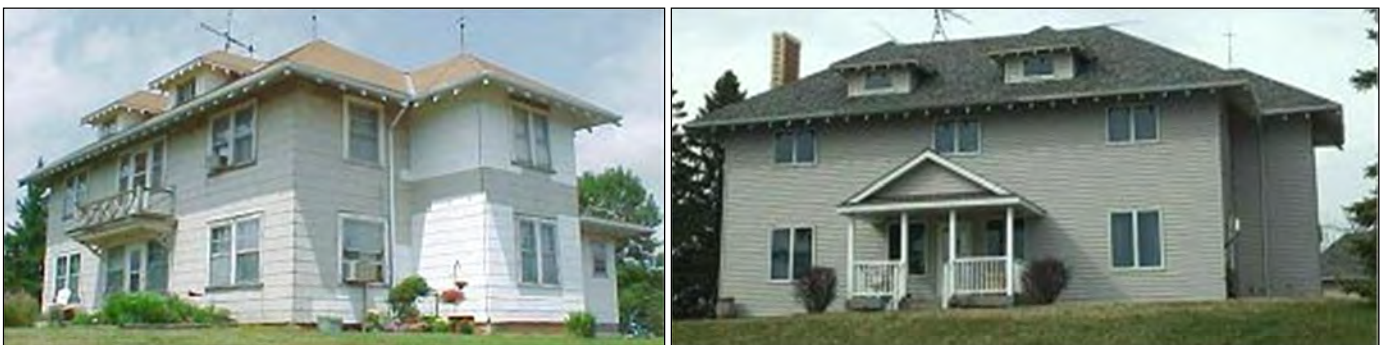
Figure 68. Escher House built circa 1915 on Long Branch Stock Farm. These two different views show the modifications this house has undergone in the modern era, from wide replacement siding and window replacements at left to the current vinyl siding, modern window inserts, and two different front porch additions. The only original elements that remain on the exterior are the roof with wide eave overhang and exposed rafter ends, and the hipped dormers on the front roof slope that have the same roof/eave treatment.
