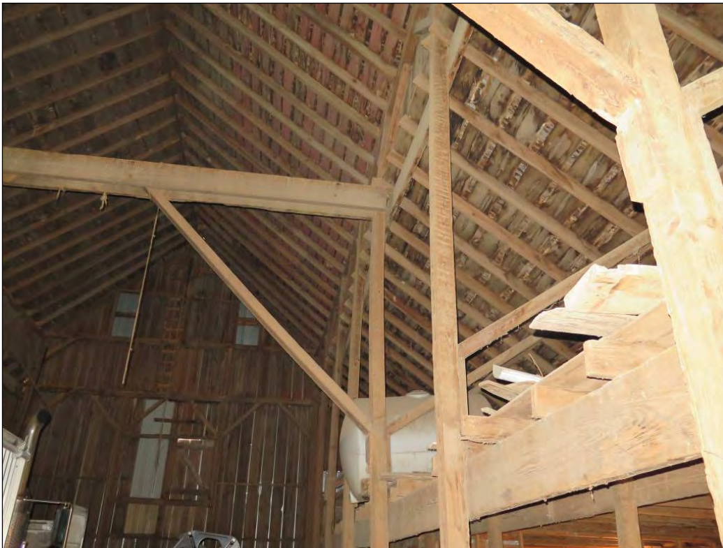
Figure 36. Interior bent and framework on the interior of the North Barn looking east. Note the two windows in the gable end of the barn that are now covered over with exterior metal siding. Photograph taken by Tallgrass Archaeology LLC, 04/13/2018.
