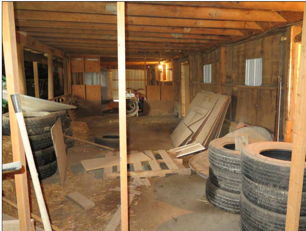
Figure 34. Interior of south section of North Barn. Note the former window openings now covered over by exterior metal siding. Photograph taken by Tallgrass Archaeology LLC, 04/13/2018.
