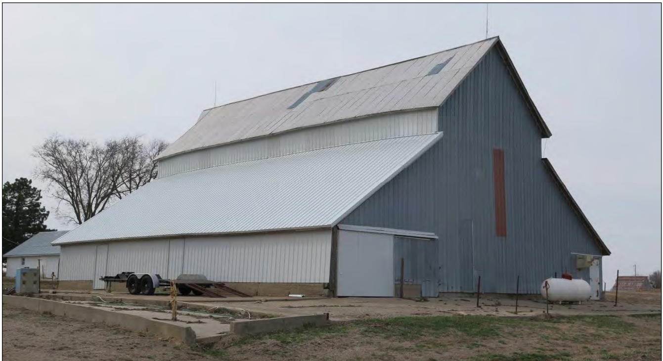
Figure 31. This circa 1910 barn is clad in modern metal siding but characterized by its distinctive monitor roof. It was originally a calving and feeding barn, but, much like the other buildings at Pleasant View, it is currently used for equipment storage.
