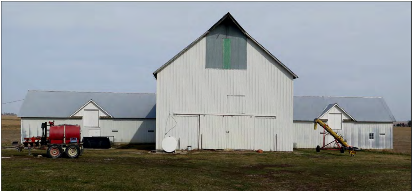
Figure 17. West elevation of the circa 1910 T-shaped South Barn. Notice the hooded hay mow and gabled dormers centered on each of the north and south wings. Photograph taken by Tallgrass Archaeology LLC, 04/12/2018.
