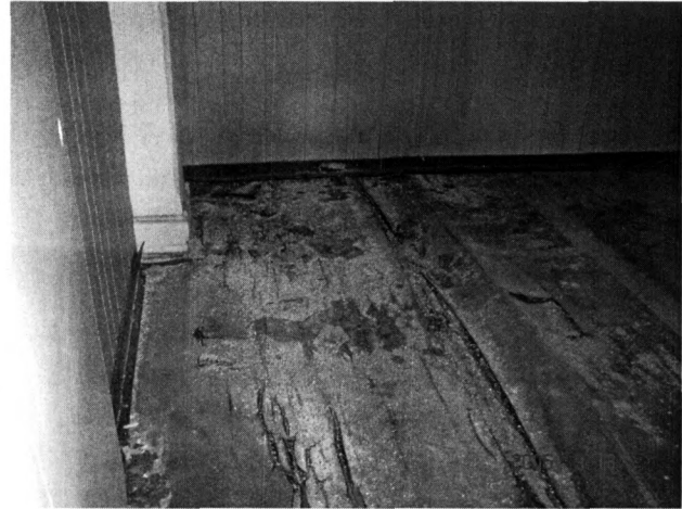
Figs. 2 & 3. Interior details of windows and floor illustrate that the Administration Building has suffered from neglect and water damage, but retains important elements of design and materials, 2008.
