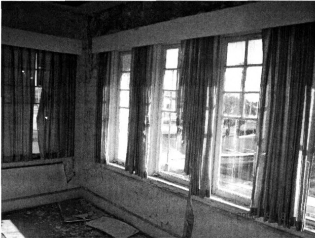
Figs. 2 & 3. Interior details of windows and floor illustrate that the Administration Building has suffered from neglect and water damage, but retains important elements of design and materials, 2008.
