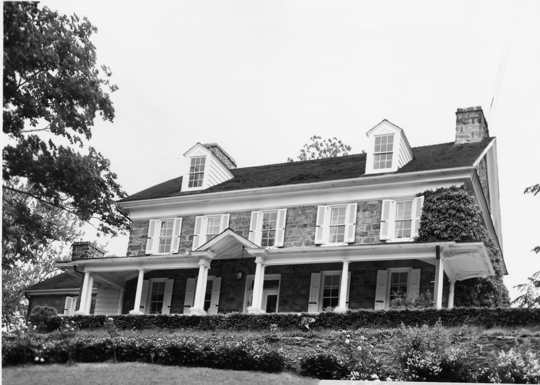
Mill Grove, south facade. (Mill Grove County Park, 1971)
