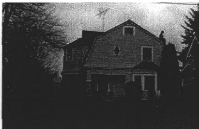
Albertson House 823 N I St. Built 1896
