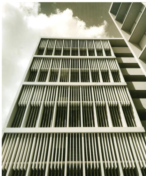
Figure No. 4: Portion of the exterior façade looking south, and detail of vestibules brise-soleils. The vertical-fins brise-soleils are set covering paired floors, with regard to the double-height vestibules right behind them. Photo to the right c. 1960-1970. Photo on the right is partial view of west elevation of the building looking south-east (2017)
