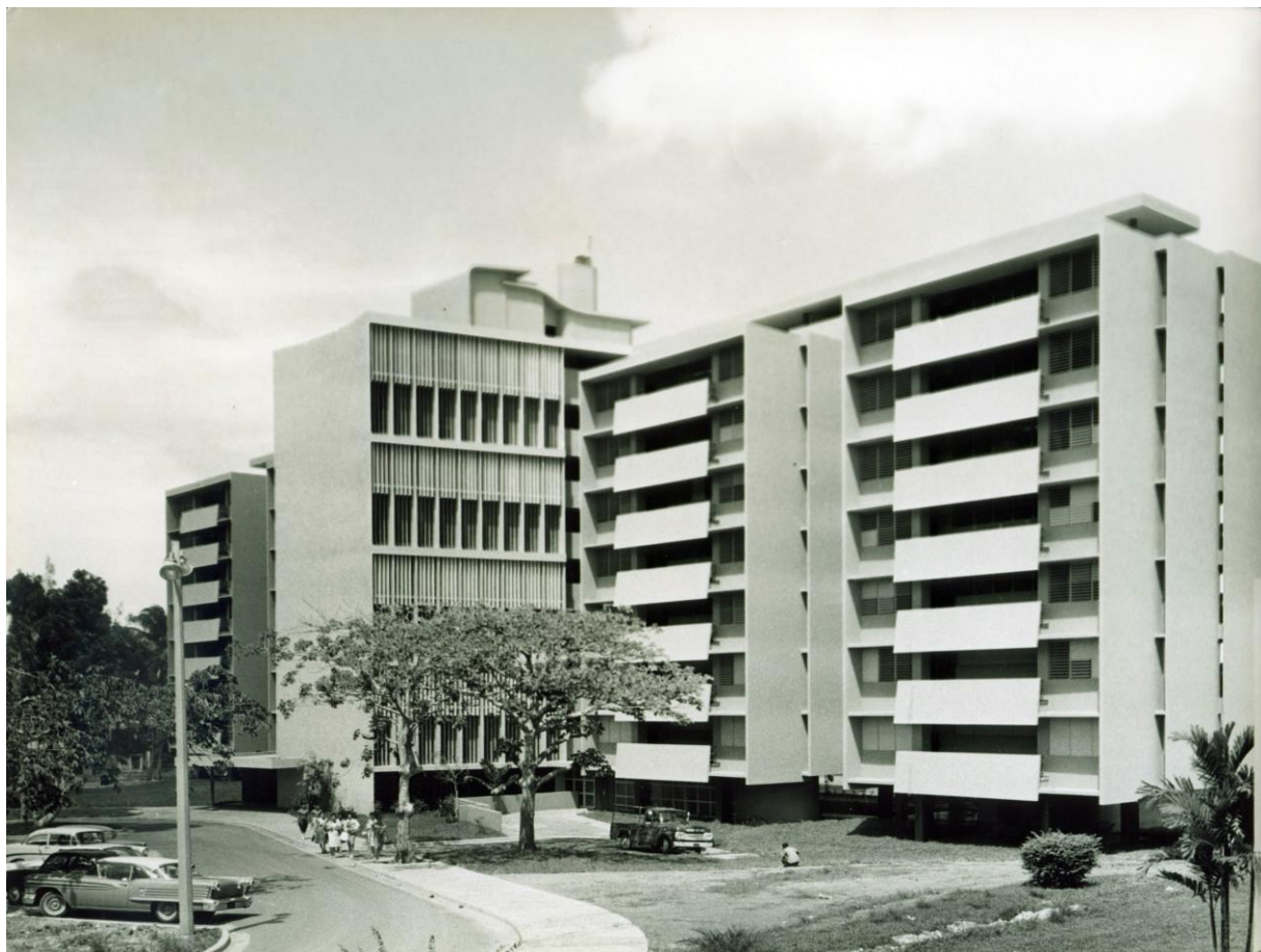
Figure No. 10: Exterior façade of complete building looking north-east. Aspect of the women’s dormitories upon initial occupation (circa 1960).
