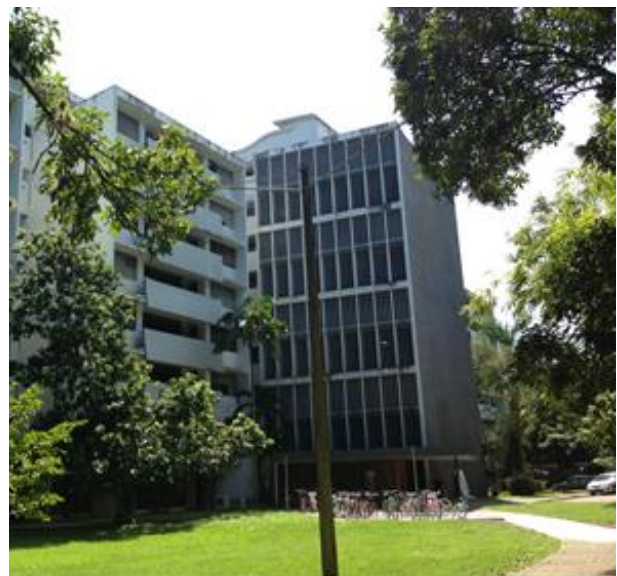
Figure No. 4: Portion of the exterior façade looking south, and detail of vestibules brise-soleils. The vertical-fins brise-soleils are set covering paired floors, with regard to the double-height vestibules right behind them. Photo to the right c. 1960-1970. Photo on the right is partial view of west elevation of the building looking south-east (2017)
