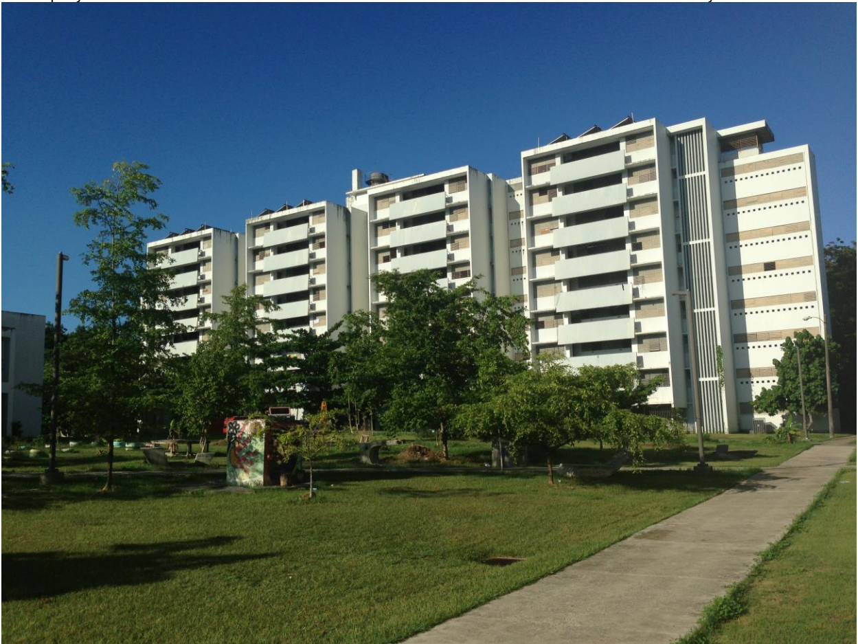
Figure No. 1: Exterior façade of complete building looking west (2017). Volumetric composition of building denotes independent dormitory volumes with intermediate gaps allowing light and ventilation on to circulation corridor (protected by operable louvers windows at East façade). Note vertical pre-fab components signaling the presence of vertical circulation (staircases) on either end of slab building.
