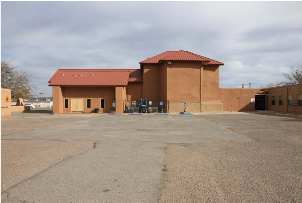
6 of 16. San Miguel Church, west (rear) elevation, with school at right, photographer facing east.
