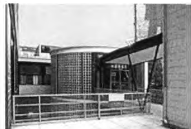
Figure 16 Drum room on another International Style Bldg.
