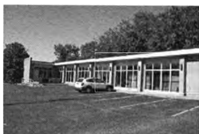
Figure 23 Potter Building 10 th Street view
