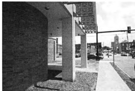
Figure 32 Milliken Building, detail of free form Wall and Piloti
