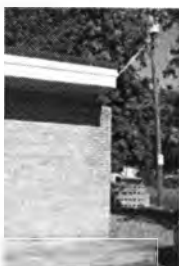
Figure 24 Potter Building Wall detail
