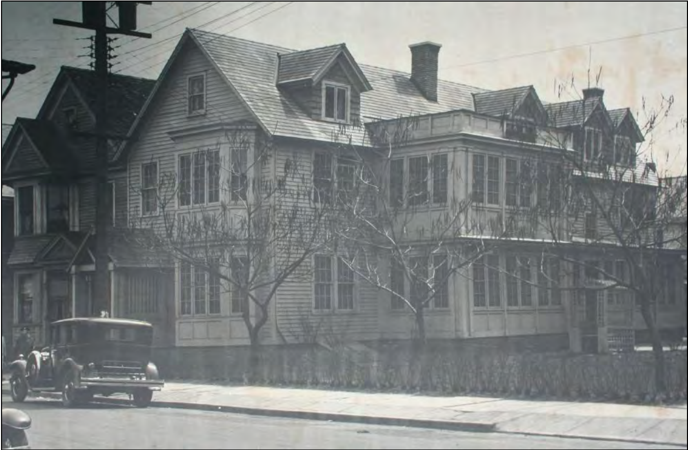
Fig.17: View of rectory, ca. 1925. Source: St. Mary's Historian's Archive.
