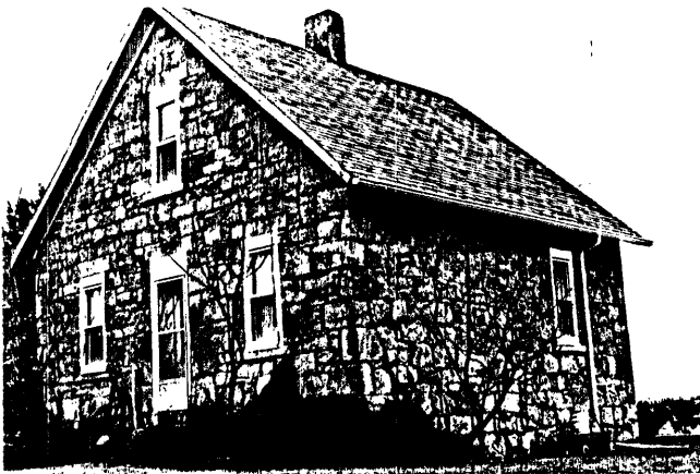
C. McDonald House (76N 28W-29) Public Facade
