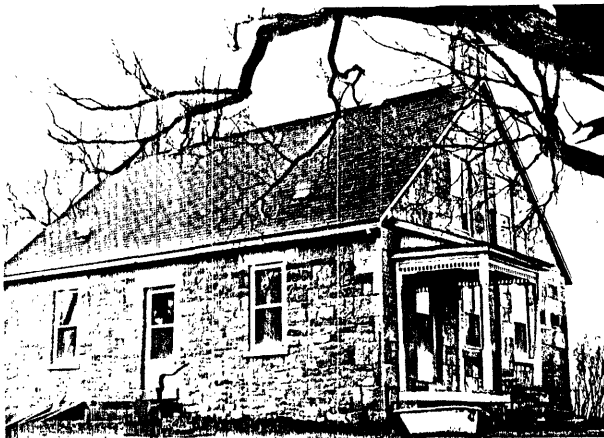
C. Early House (76N 29W-11) One Story Raised Basement
