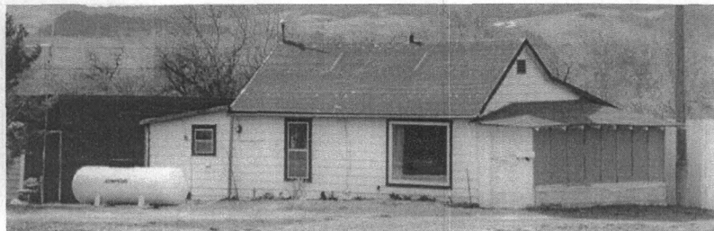
The cabin in 2000, prior to restoration.
