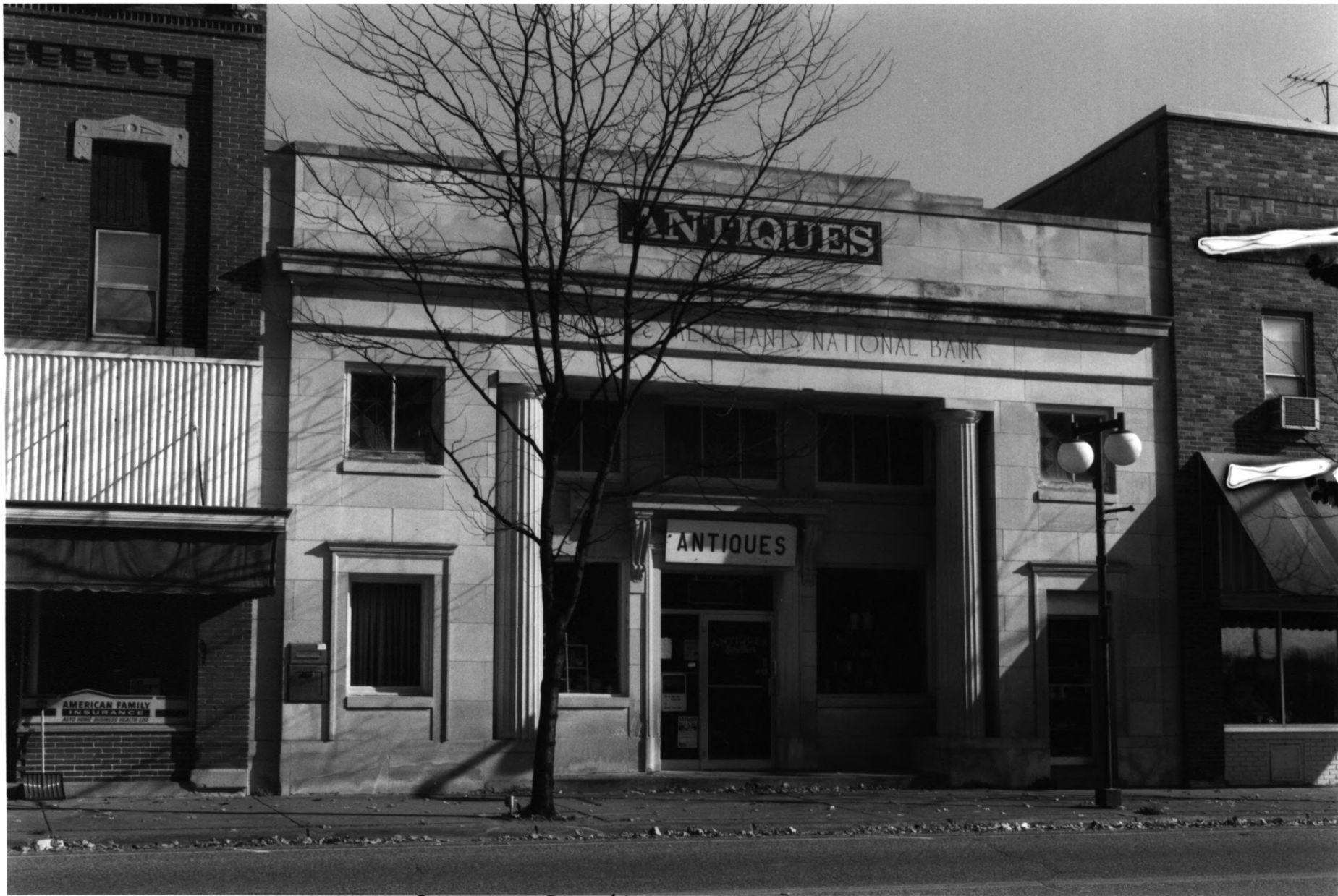
Farmers and Merchants National Bank #5 Cannon Falls Commercial Historic District Goodhue Co., Minn 013455-25
