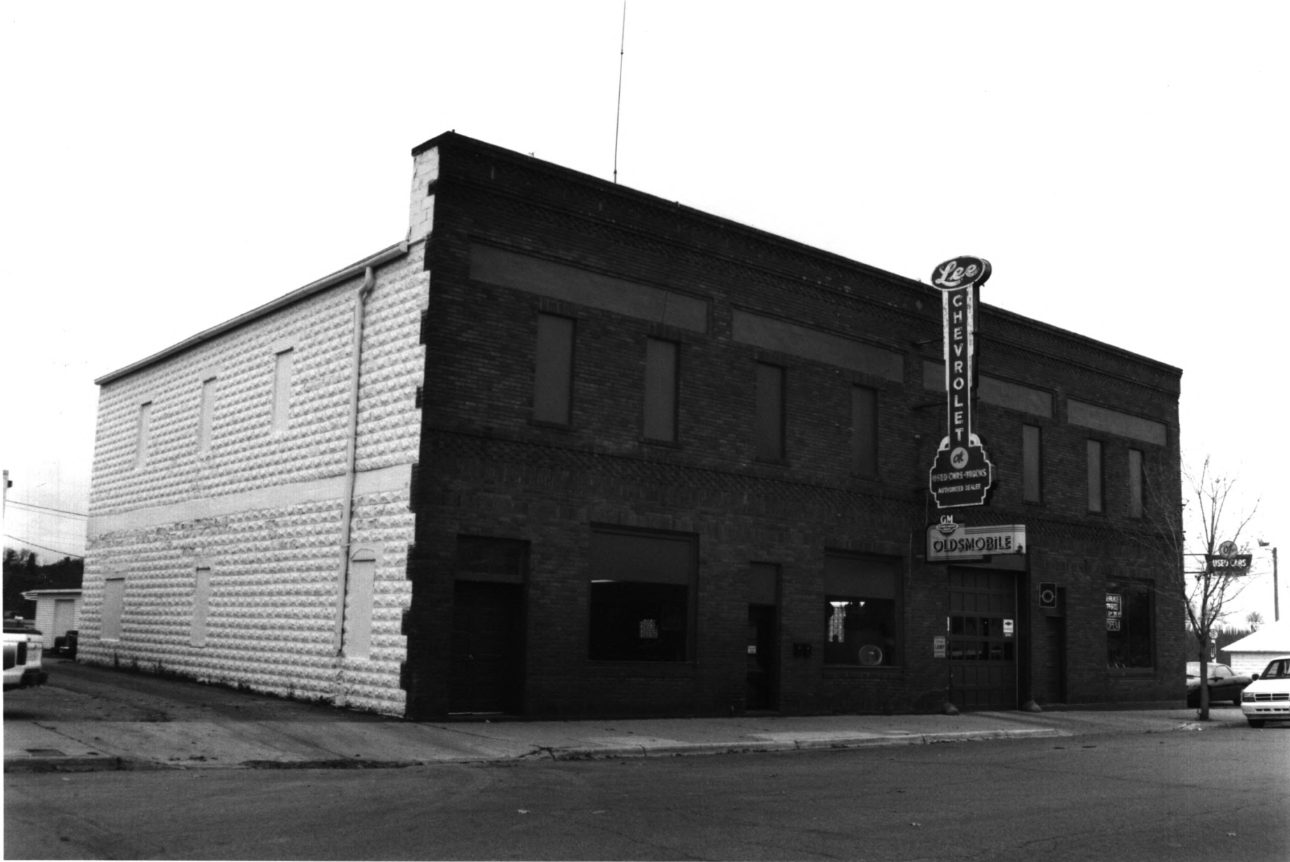
Kruse Garage #29 Cannon Falls Commercial Historic District Goodhue Co., MN 013457-1
