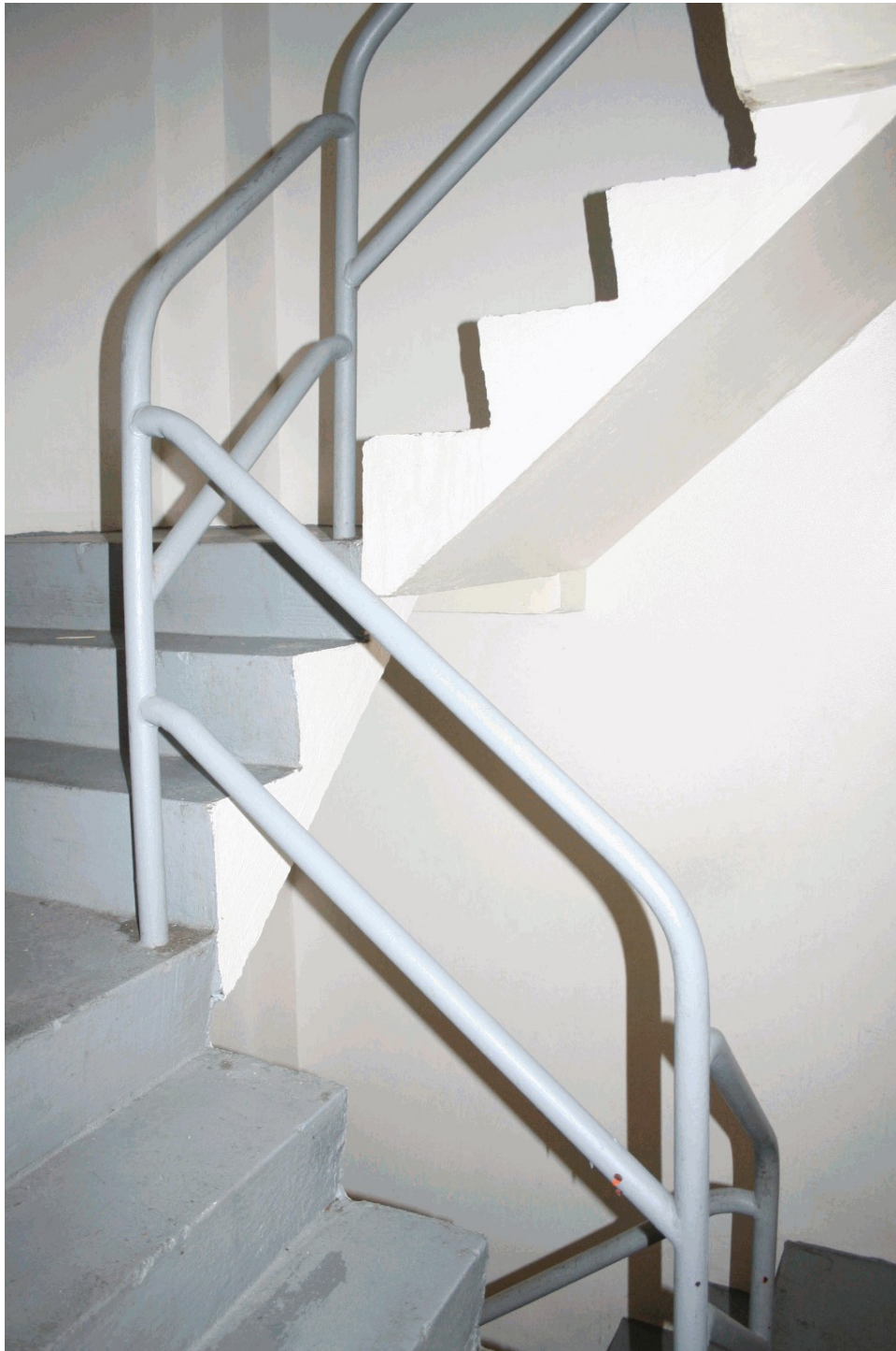
15 of 18 Stairway, typical, looking southwest
