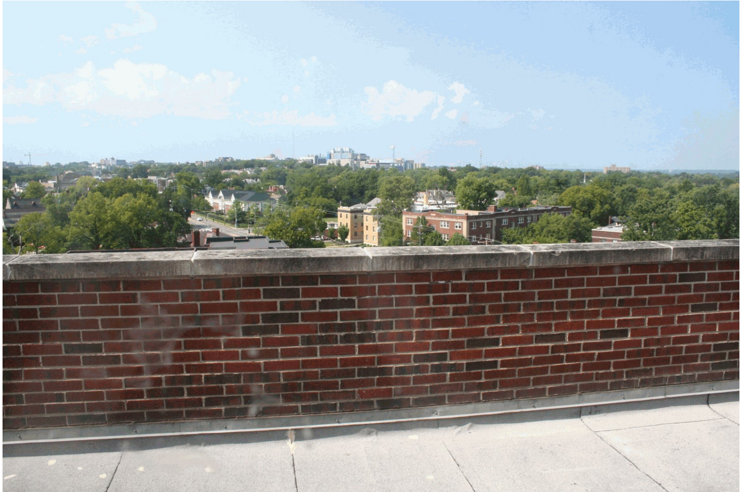
18 of 18 View from roof terrace, looking southwest
