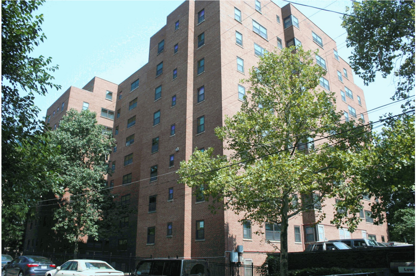
3 of 18 Rear (east) and south (side) elevations, looking north
