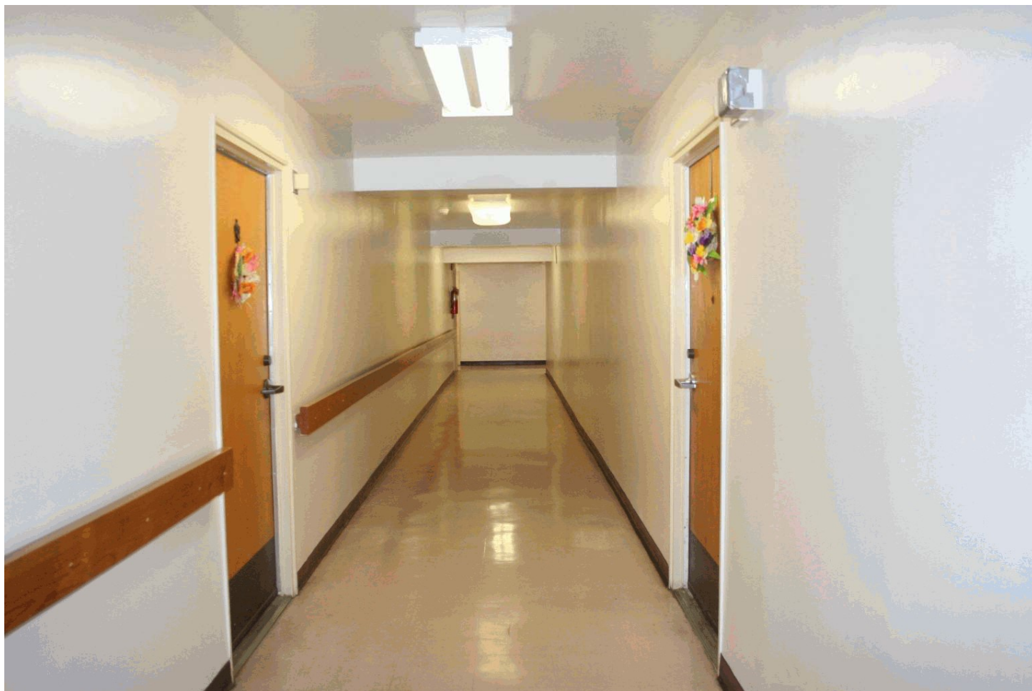
11 of 18 Corridor, typical, looking southeast
