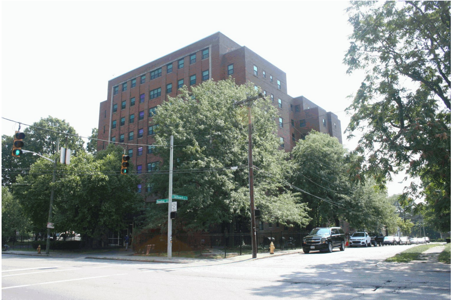
1 of 18 Front (west) and south (side) elevations, looking east
