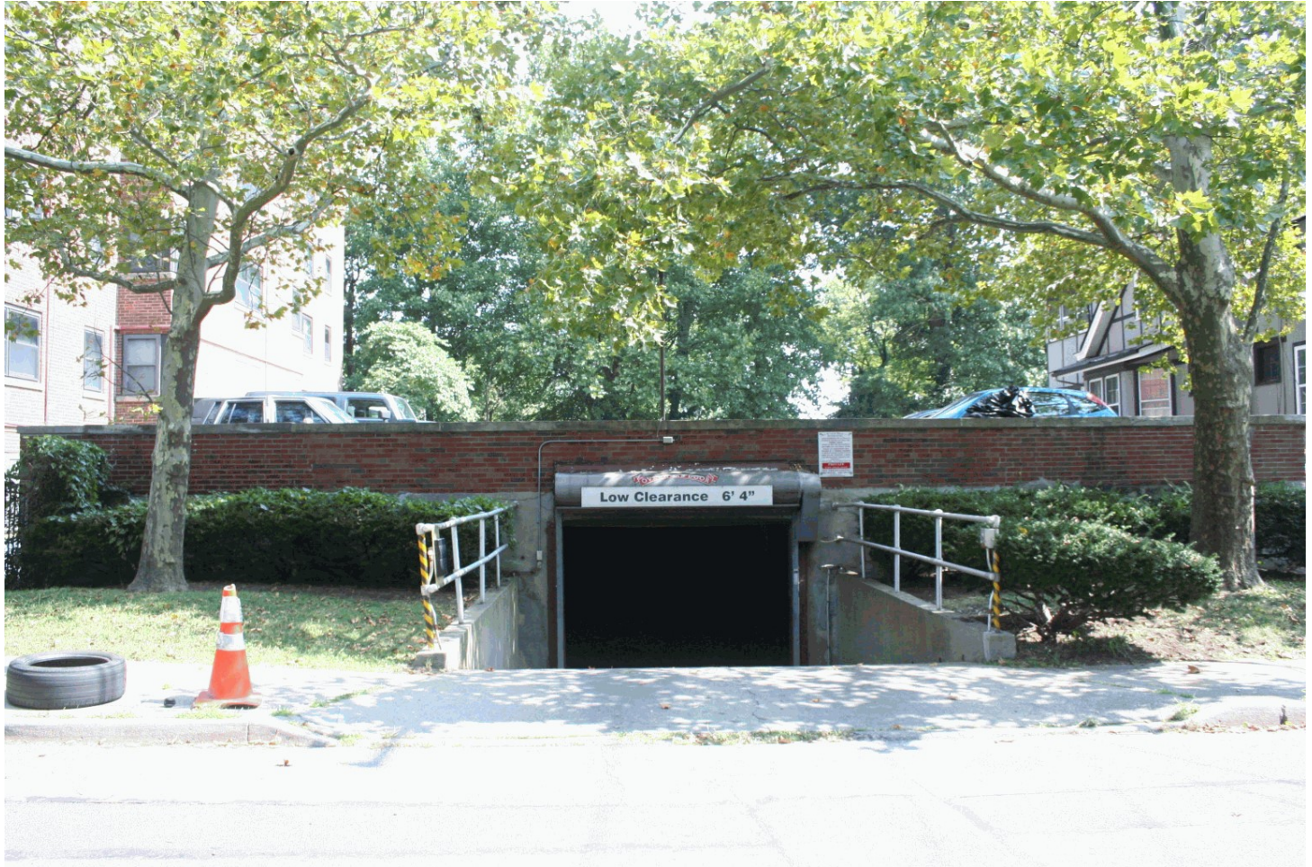
5 of 18 View of garage, looking northeast
