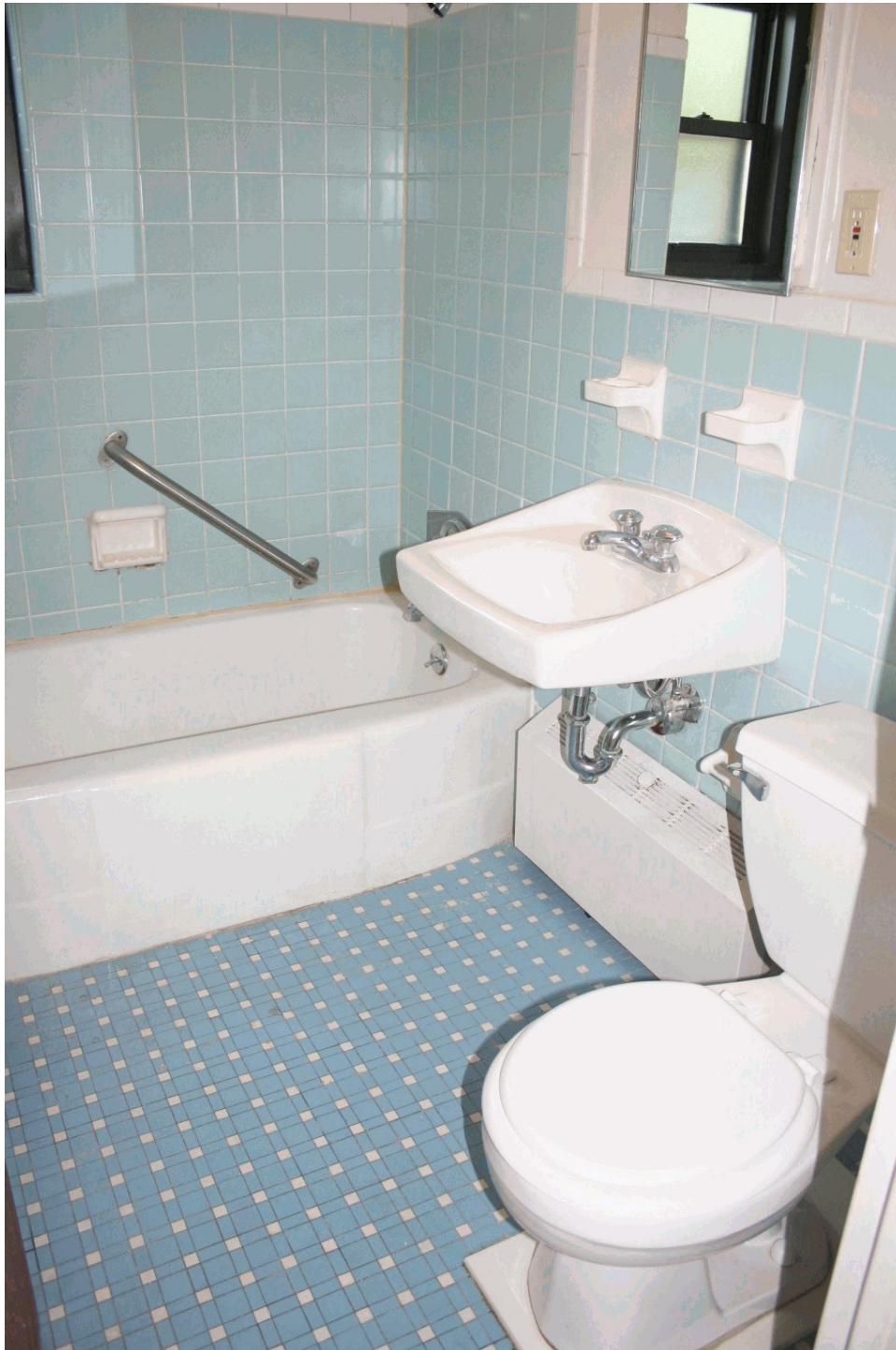
14 of 18 Apartment Bathroom, typical, looking west
