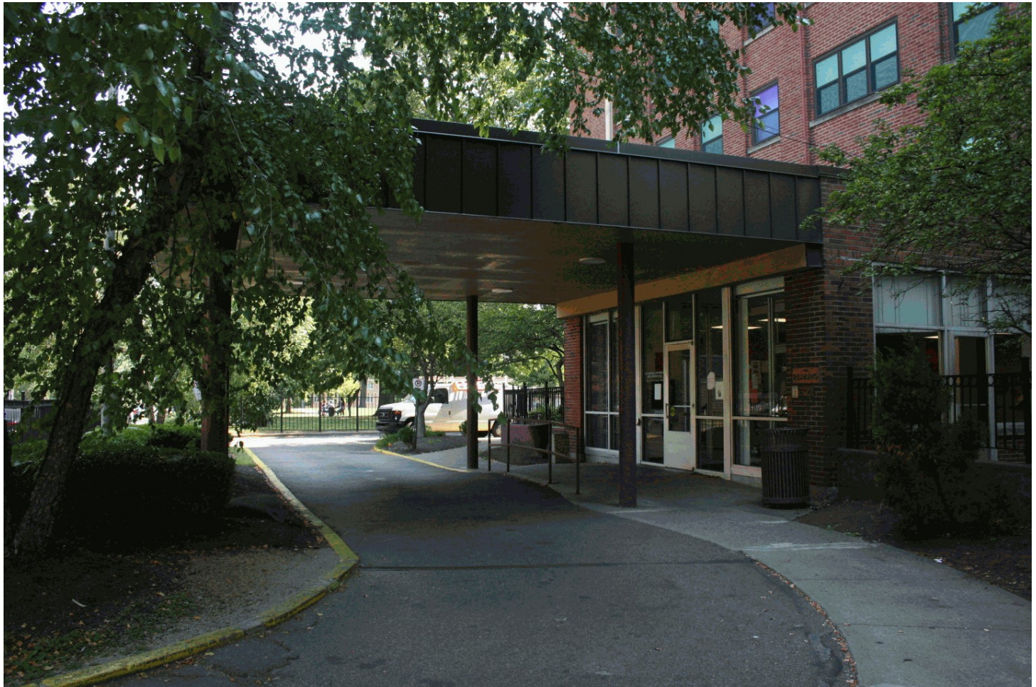
7 of 18 Front driveway, looking northeast
