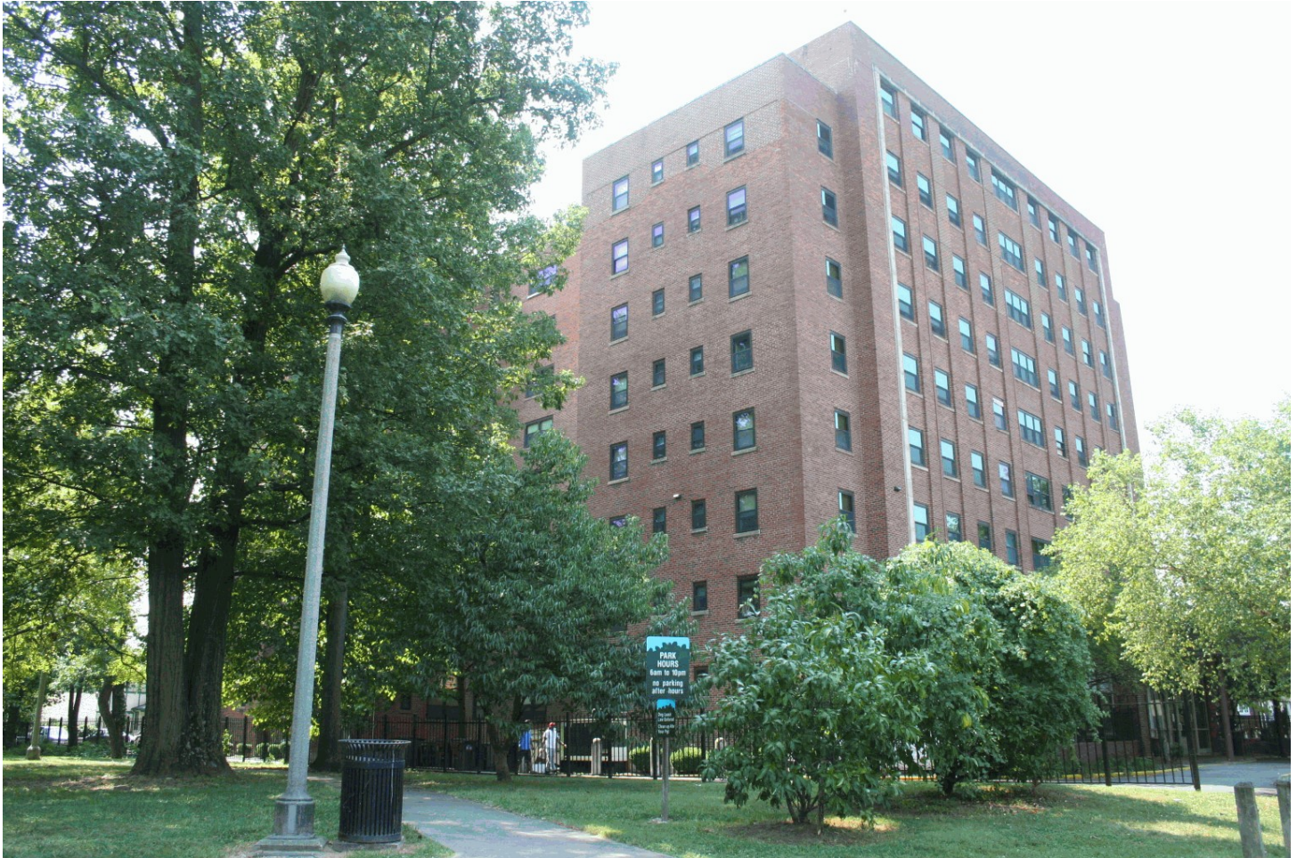
2 of 18 Front (west) and north (side) elevations, looking south
