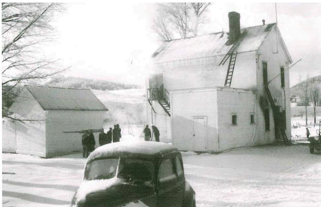
Figure 3. View looking west during the fire in 1951. The flat-roofed addition housed a woodshed and chemical toilets. Courtesy of the Underhill Historical Society.
