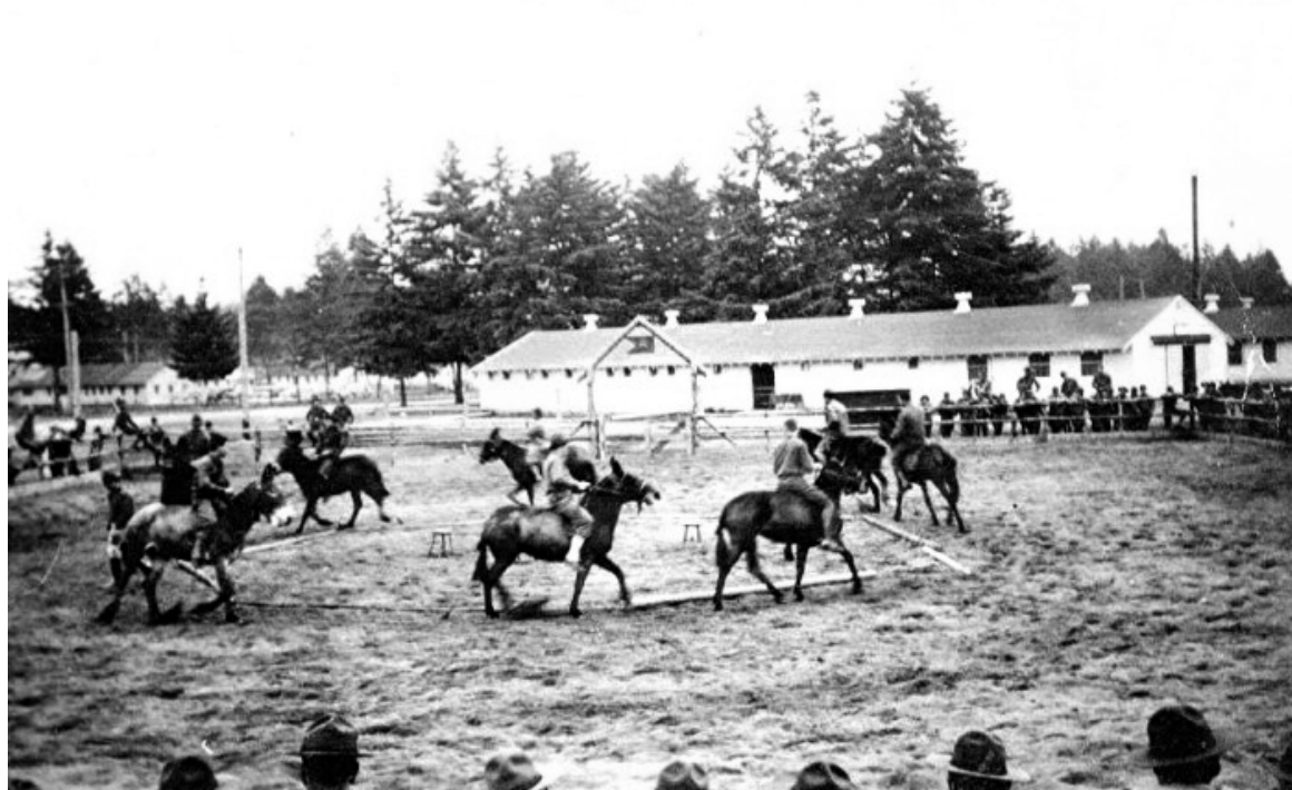
Figure 15. 98 th Field Artillery musical chairs with mules, Fort Lewis, Washington, 1942. Series 700-486 ward in background identical to Fort Ord's Wards A and B. Number of roof ventilators could vary: six here, five at Fort Ord. Photo: R.B. Lawson Collection. From Krenzelok.
