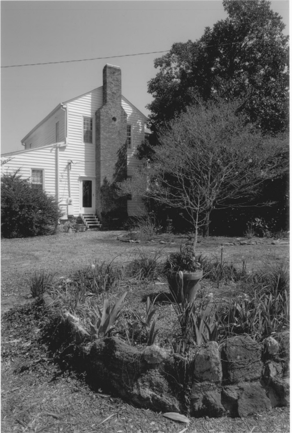
Martin and Lucretia Stamper House Talbot County, Georgia Photograph 5 of 19
