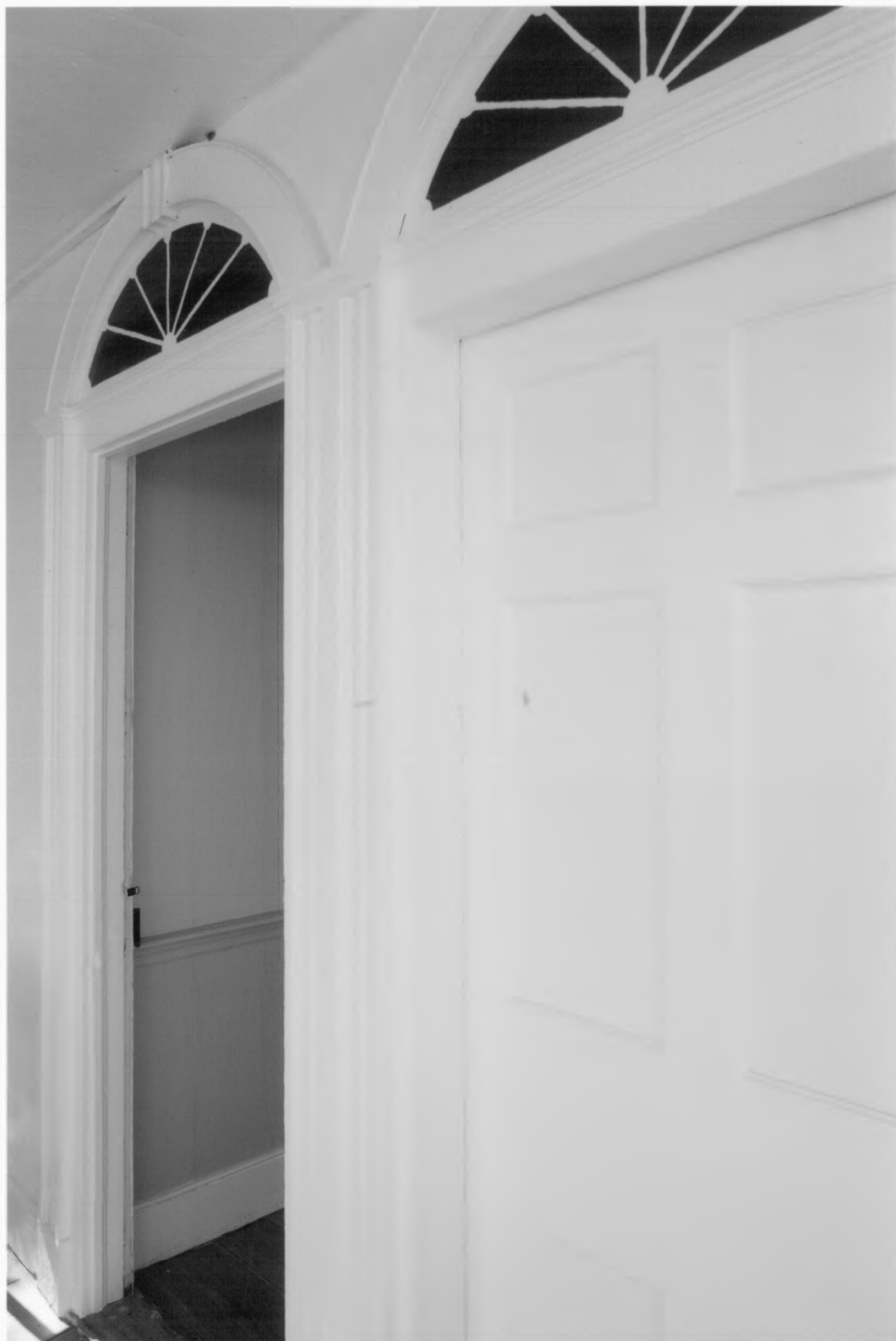
Martin and Lucretia Stamper House Talbot County, Georgia Photograph 9 of 19
