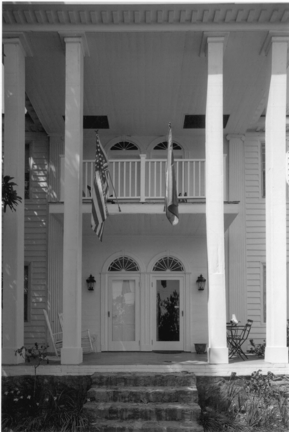
Martin and Lucretia Stamper House Talbot County, Georgia Photograph 8 of 19
