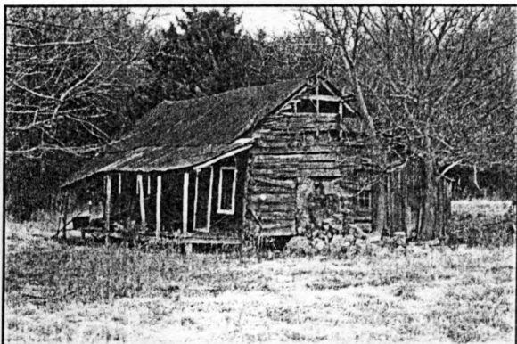
6. Log House, oblique, camera facing NE 7. Photo #10
