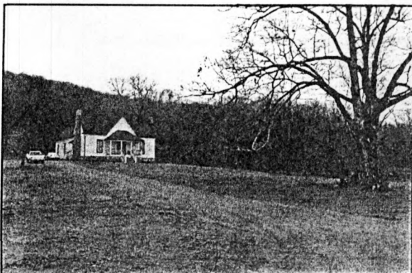
6. Site, oblique, camera facing NE 7. Photo #8
