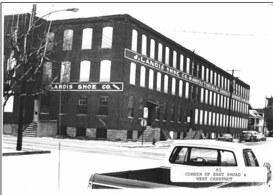
Figure 19 - Landis Shoe Company (1906), Palmyra, Lebanon County, PA, CRGIS .
