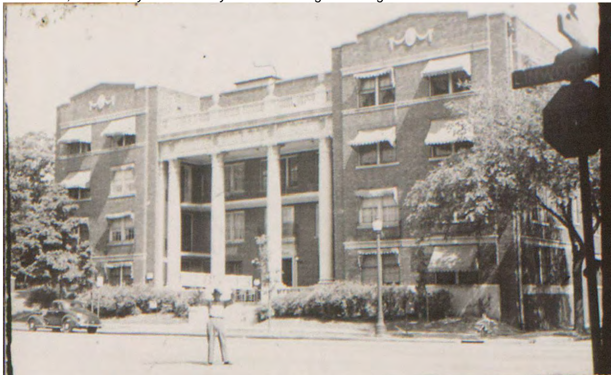
Figure 7: Gotham Apartments, 1940 Tax Assessor Photograph. Source: Missouri Valley Special Collections, Kansas City Public Library via Missouri Digital Heritage.
