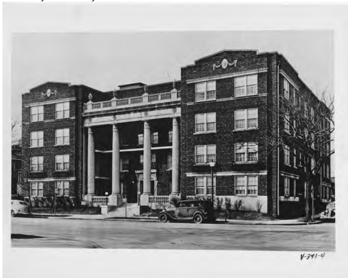
Figure 5: Gotham Apartments, historic photograph, c. 1920s. Source: Missouri Valley Special Collections, Kansas City Public Library.
