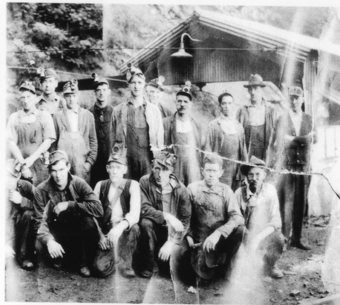
Panorama detail showing headhouse in background. Notice extended beam that supports the roof. This was removed after the mine closed causing the roof to collapse at that corner (see modern photo #4).
