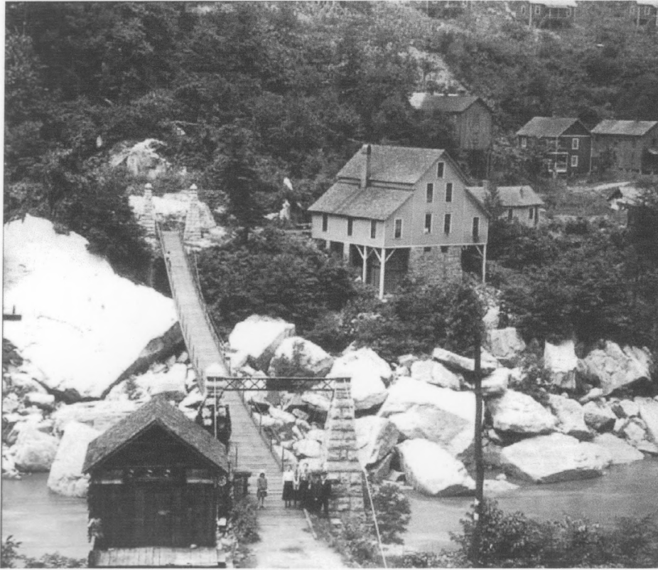
Views of the Nuttallburg Suspension Bridge shortly after completion, looking towards South Nuttall, 1899 (C&O Historical Magazine)
