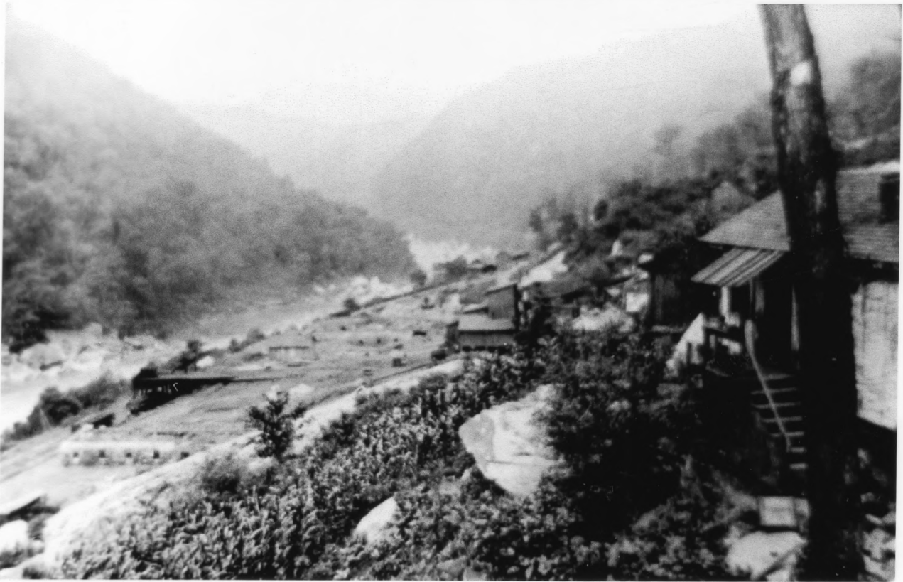
Original Nuttallburg tipple, wooden structure with tower in middle of frame. Banks of coke ovens lie perpendicular to the river. (NERI 315)
