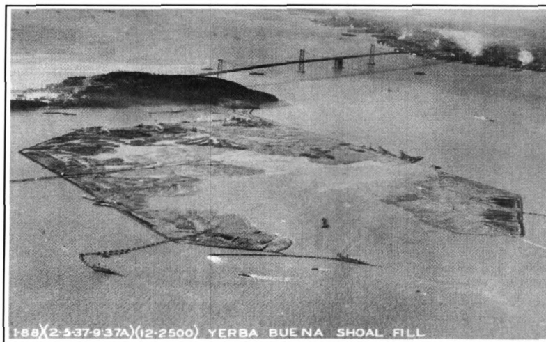
Figure 4. Filling of Yerba Buena Shoals, showing construction of the permanent building (left) February 5, 1937. [Unit 2, Shelf B, Folder Treasure Island, Construction and Plans, Treasure Island Museum Collection]
