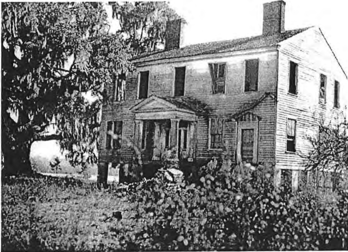
Figure 4. Gregory House, on original site on west side of the Apalachicola River, 1936.
