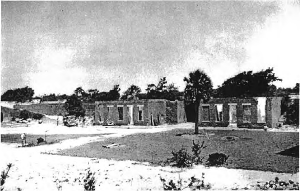
Figure 6. Fort Clinch during restoration, ca. 1937
