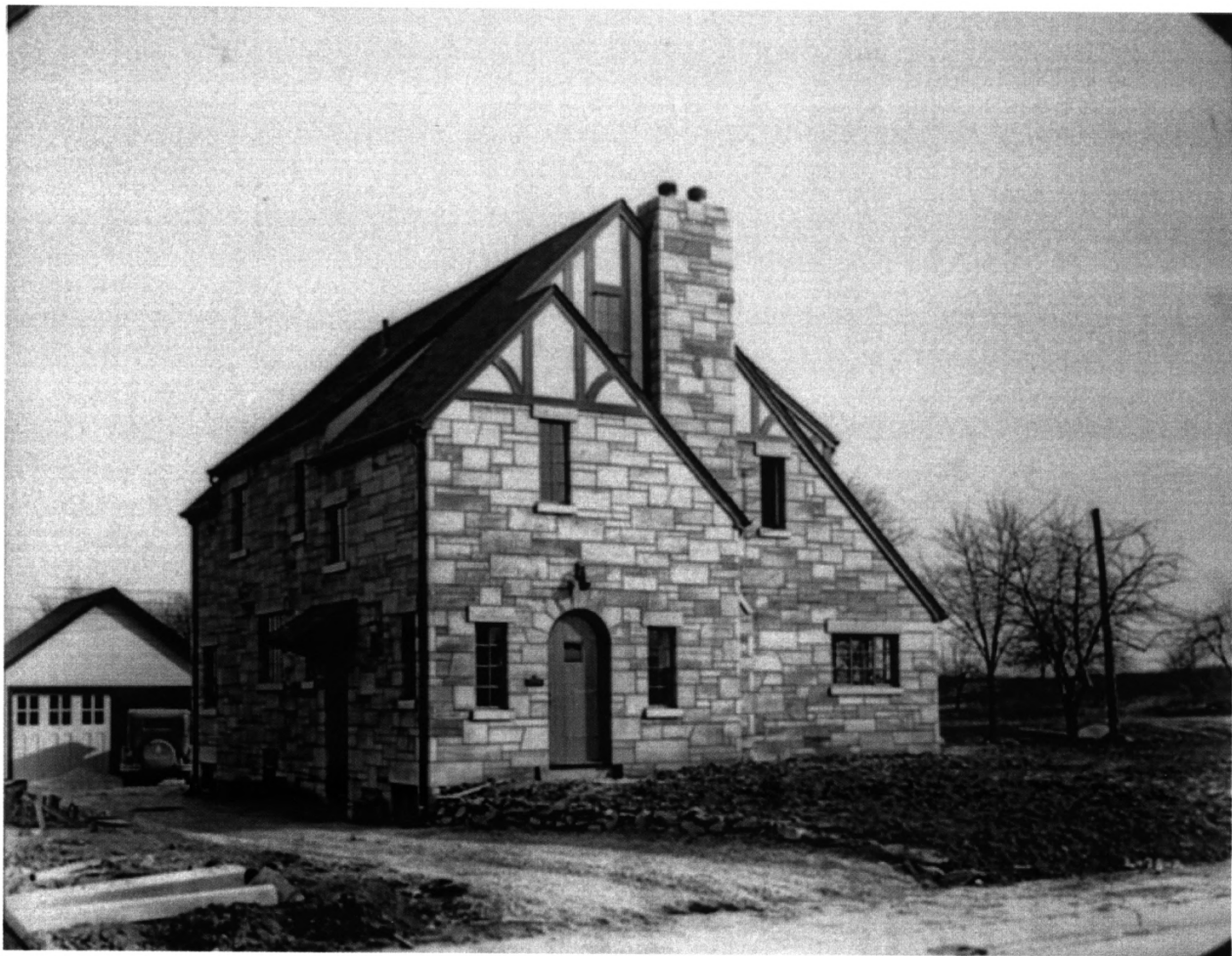
Alfred and Kathleen Evens House • 727 S. Jordan Ave. (52) c1930 camera facing southeast
