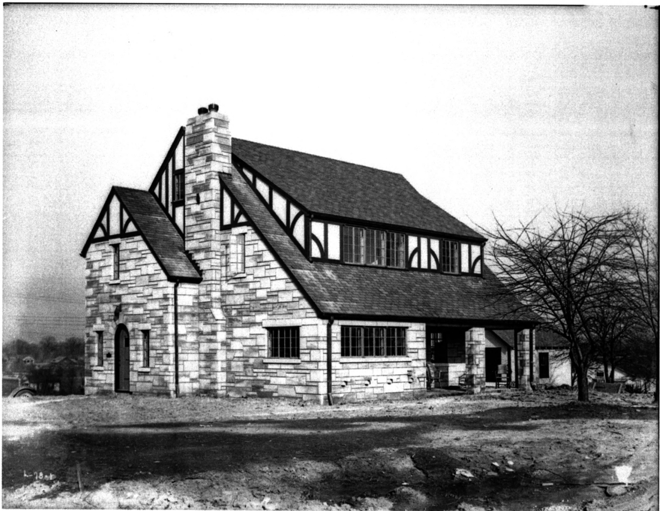
Alfred and Kathleen Evens House • 727 S. Jordan Ave. (52 c1930 camera facing northeast
