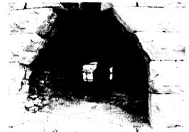
At one time, a brick wall existed between the outer opening and the inner chamber opening. This wall has partially collapsed. The brick wall was most intact in the east kiln. The west kiln appears to have extended the inner brickwork out to be integrated directly into the outer stone masonry wall. The eastern kiln brickwork ended between the inner and outer walls.
