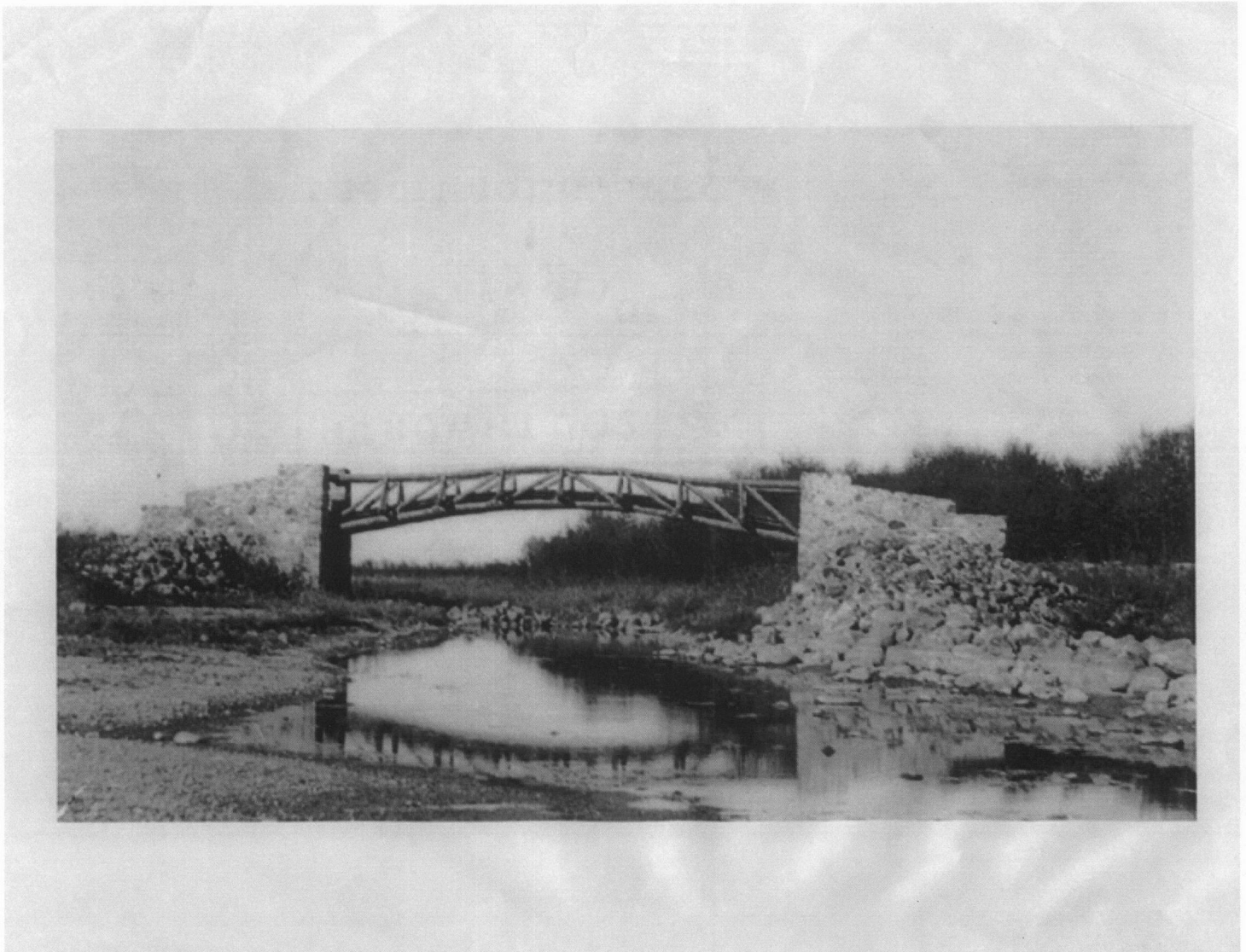
Nonextant bridge at Mini-Wakan State Park, c. 1935. The bridge was constructed to the west of the picnic shelter. (Photo courtesy of Juliana Mayne, Mini-Wakan Committee.)
