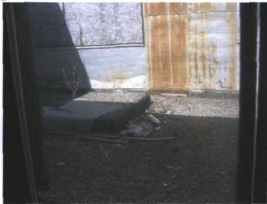
Skylight Courtyard (from Second Floor)
