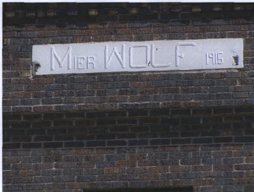
Building Identification Plaque on Facade
