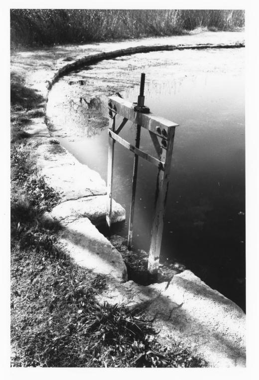
(3) Rattlesnake Springs Pond, limestone block wall of east side of pond, showing iron headgate,
