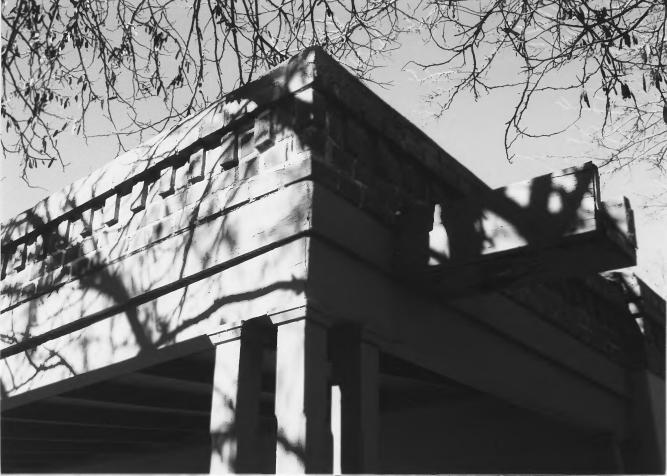
Ranger's Residence, NPS Bldg #22, (C), SE corner of portal showing chamfered box columns with Doric caps, wooden entablature, brick denticulated cornice, and wooden canale.
