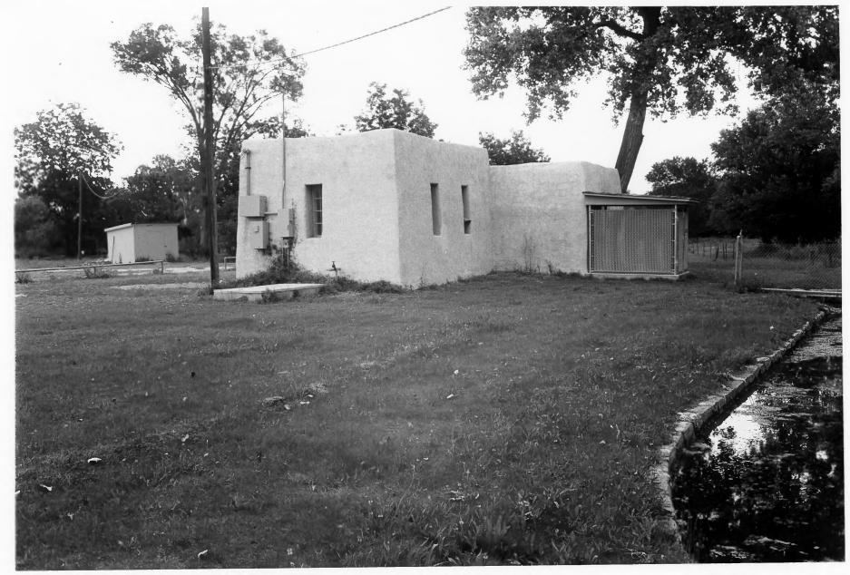
(2) Pump House, NPS Bldg #20, (C) rear looking NE showing 1986 addition to house chlorine tank.
