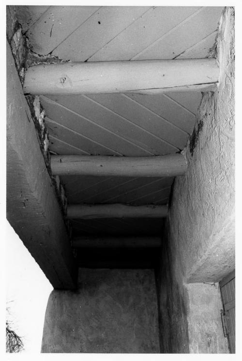
(2) Pump House, NPS Bldg #20, (C), ceiling of recessed entrance or narthex, showing <u>vigas</u>, planks laid in herringbone pattern, adzed lintel.
