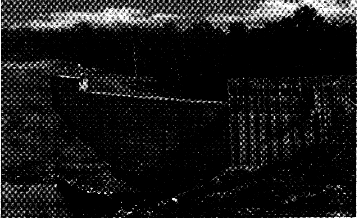
60 ACRE RESERVOIR, 1 MILE EAST OF ADA, OKLA.
