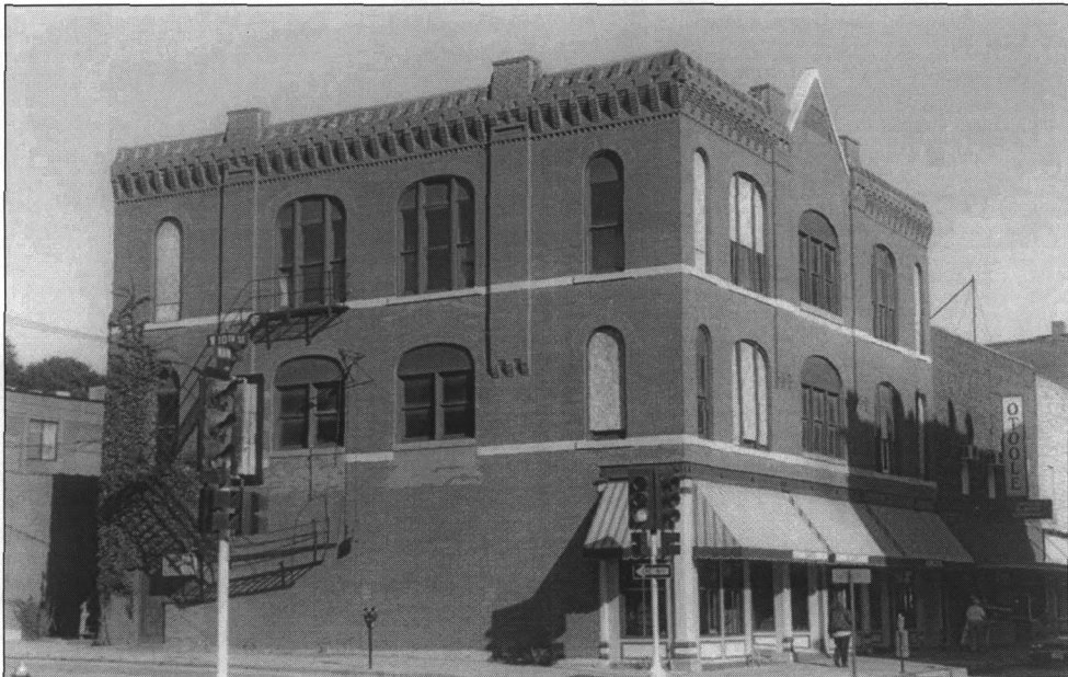
Figure 5: 1005 Main, view north (photo by J. Jacobsen, August 2004)
