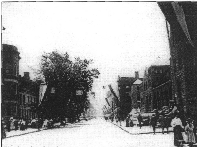
Figure 31: Main Street, viewed south from West 12 th Street, c.1910 (Center For Dubuque History, Loras College)
