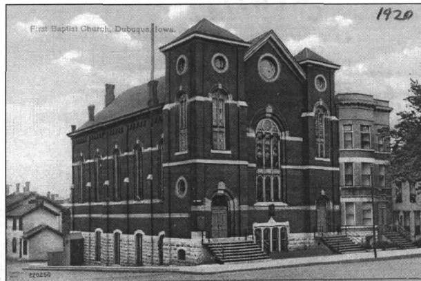
Figure 29: First Baptist Church, 13 th and Main, view southwest, postcard view, c.1920 (non-extant) (Center for Dubuque History, Loras College)
