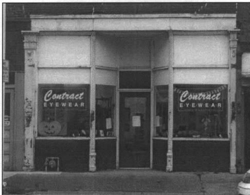
Figure 2: Storefront detail, surviving cast iron front, 1066-68 Main (photo by J. Jacobsen, November 2002, view east)
