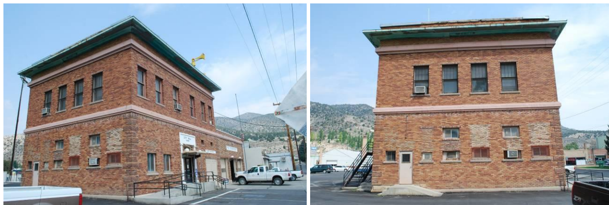
Photograph 6 and 7: East façade and south elevation, looking northwest (left), and south elevation, looking north (right) (NVSHPO, 2015).
