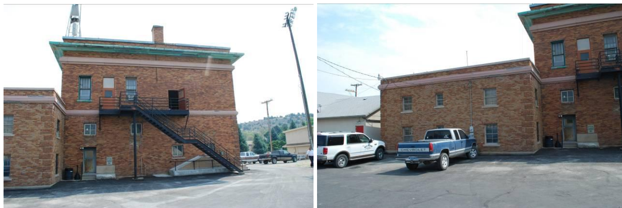
Photograph 4 and 5: Rear elevation looking east (NVSHPO, 2015).
