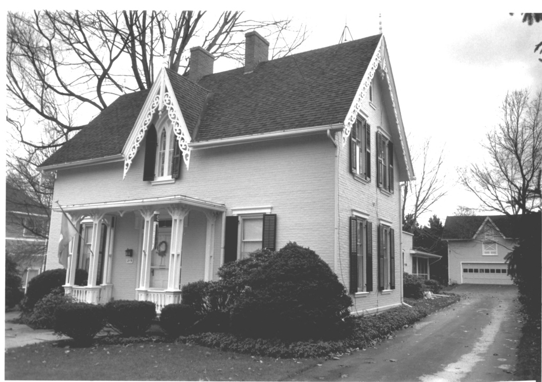
18. Marshall Historic District Marshall, Michigan Chastian-Mann-Foster House Photo: Susan Collins, 1990
