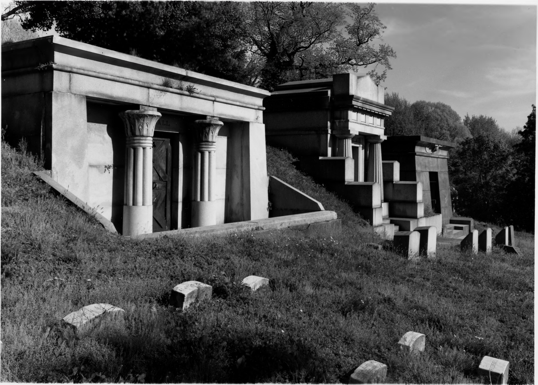
Fig. 13 Laurel Hill Cemetery Philadelphia, Pennsylvania Ball, Lane and Dolan mausoleums, 1997 (J. Boucher)
