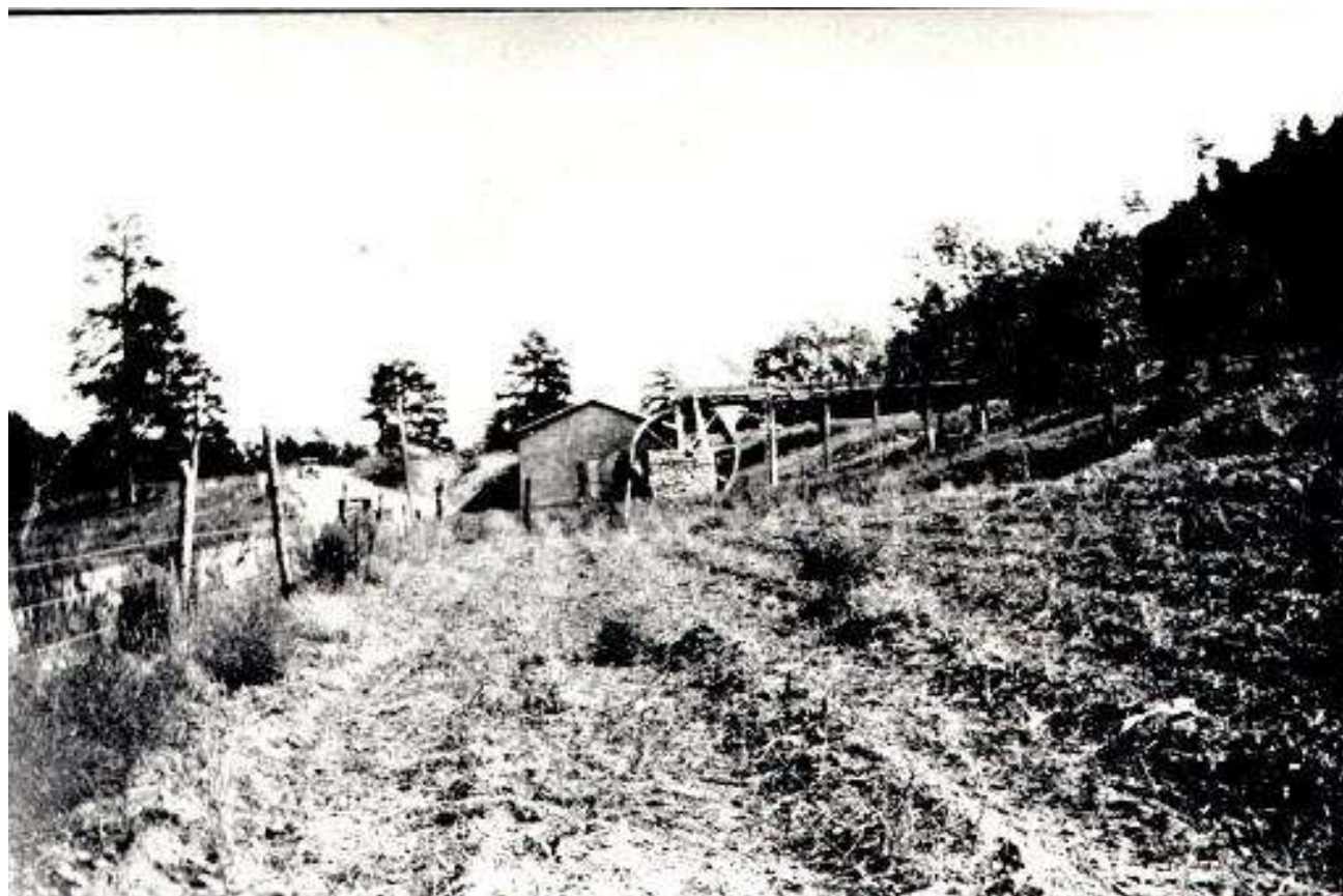
Figure 6 Vintage Photo 6 of 16, circa 1920, Old Dowlin Mill, camera facing east
