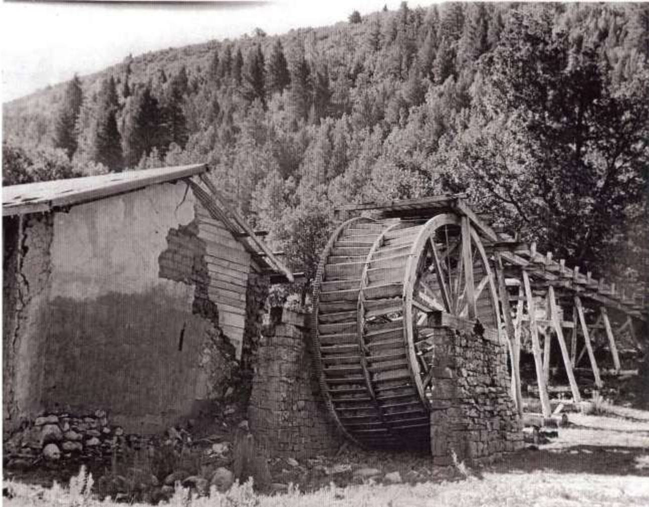
Figure 9 Vintage Photo 9 of 16, circa 1938, deteriorating condition of building and water wheel, camera facing southeast
