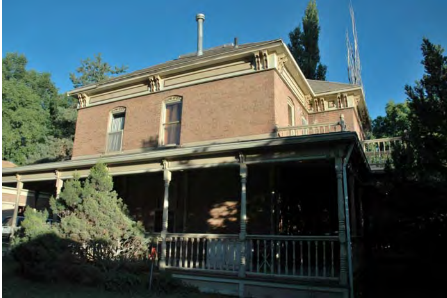
Photograph 2 of 10 North and west elevations of Wayman House. Camera facing south.
