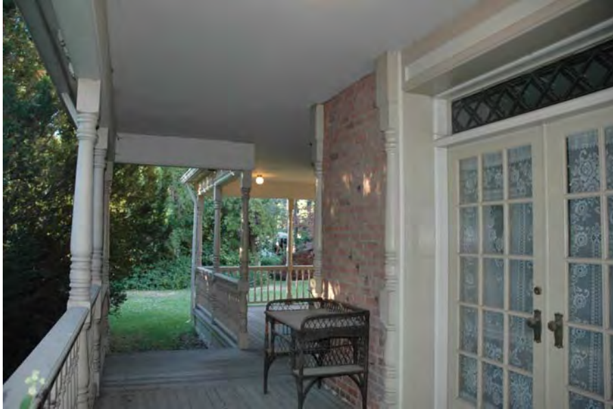
Photograph 4 of 10 West elevation of Wayman House, south entrance detail. Camera facing north.
