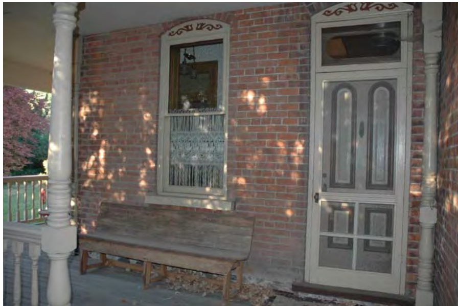
Photograph 3 of 10 West elevation of Wayman House, porch detail. Camera facing northeast.
