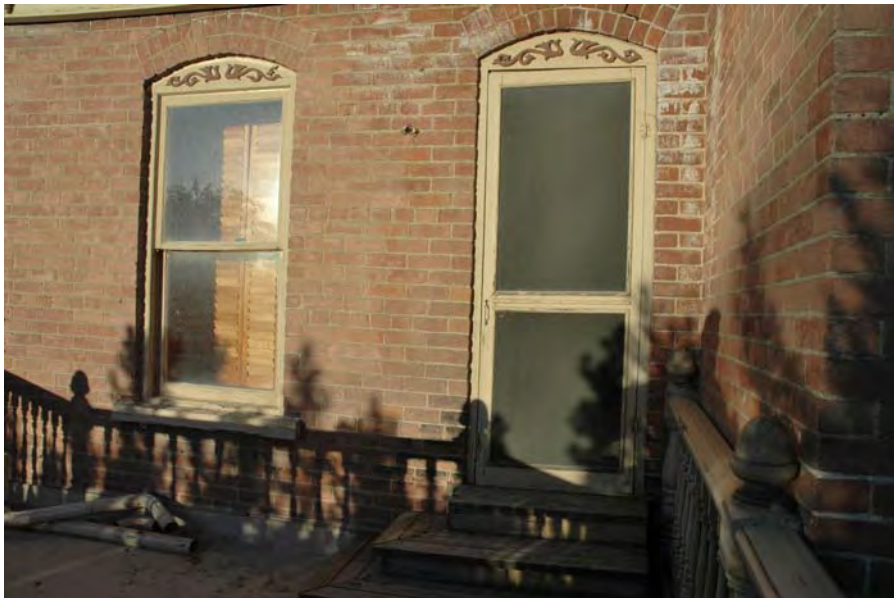
Photograph 5 of 10 West elevation of Wayman House, balcony detail. Camera facing northeast.
