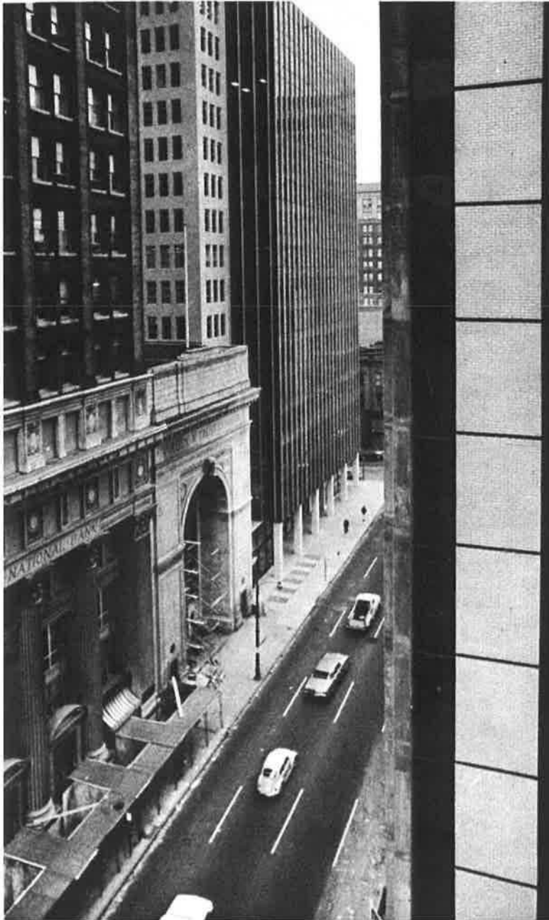
Historic Photo 2: East Main Street, Facing West, Circa 1967. Fidelity Building on Right, Ross Building in Center. Unknown Photographer. Source: Sanford 1975.
