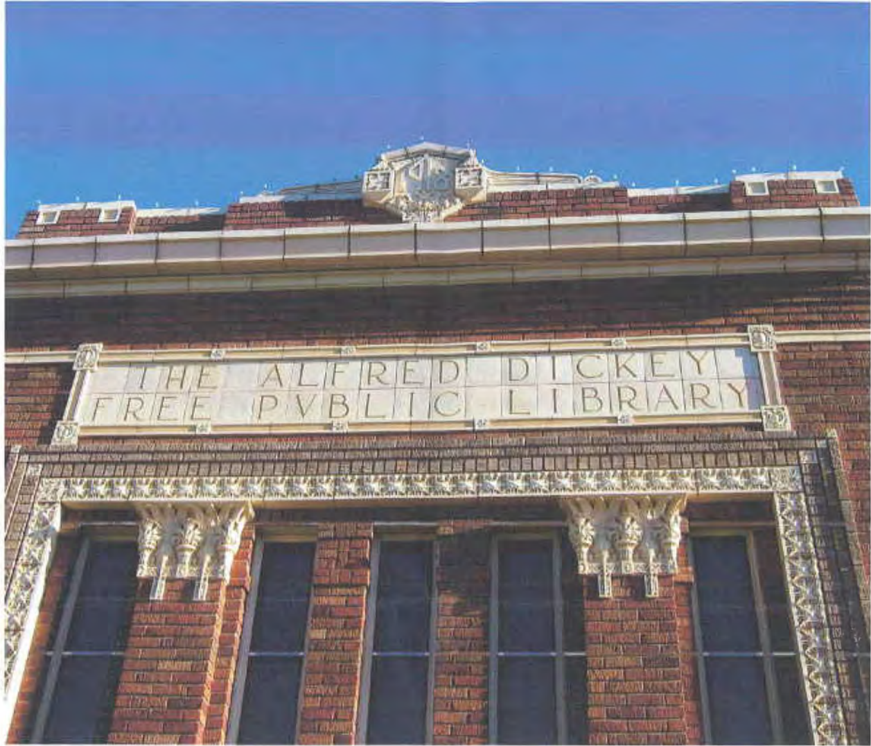
Front plaque with correct name of library. Photo provided by Bill Kennedy, Development Director, James River Valley Library System. Provided in January 2019.
