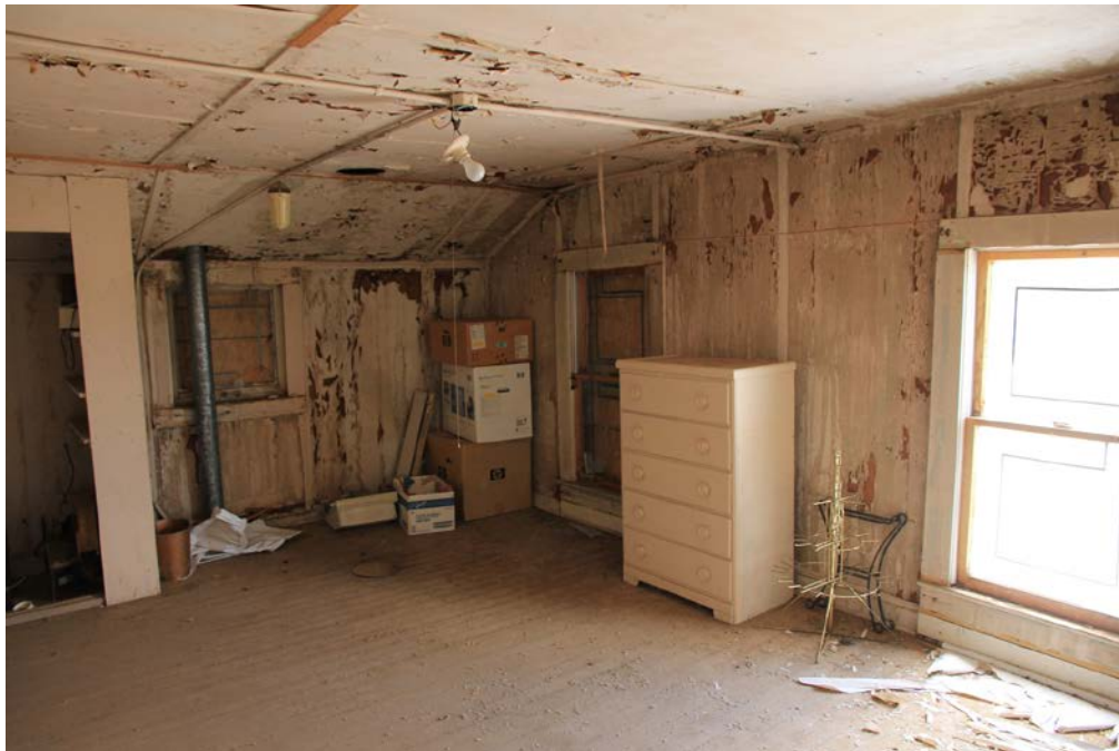
16. Interior, second floor, bedroom, photographer facing northeast.
