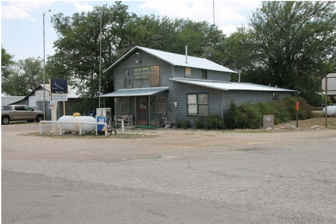
3. Main and north sides, photographer facing southwest.
