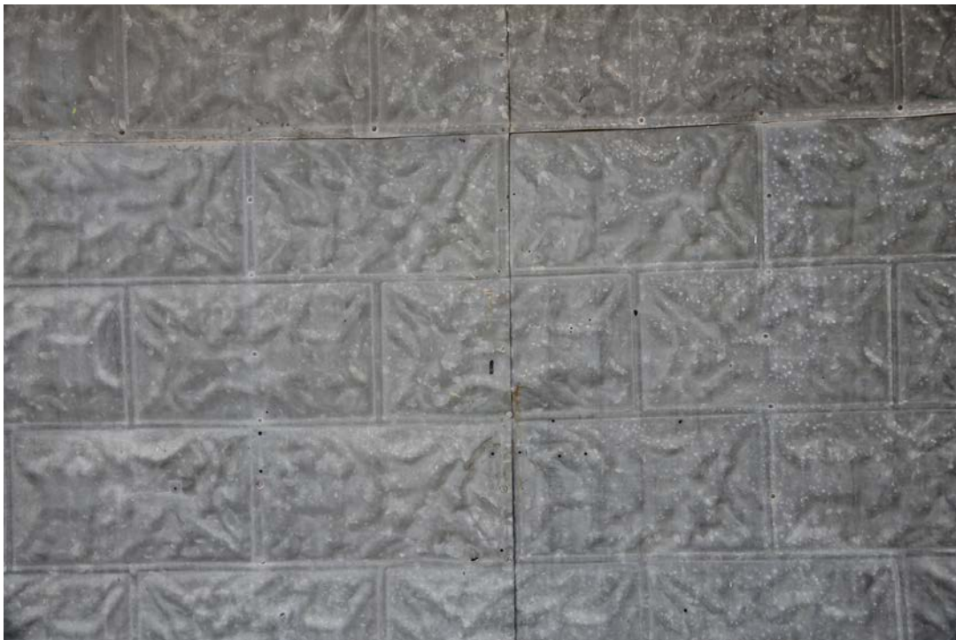
6. South side, detail of rock-faced sheet metal siding, photographer facing north.
