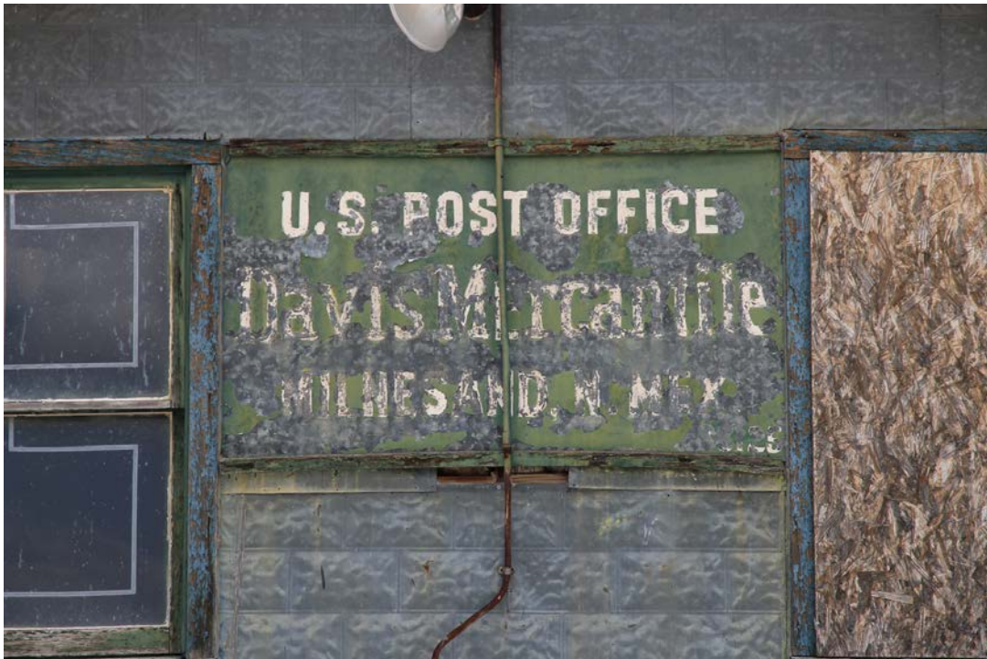
2. Main façade, detail of second-floor sign, photographer facing west.
