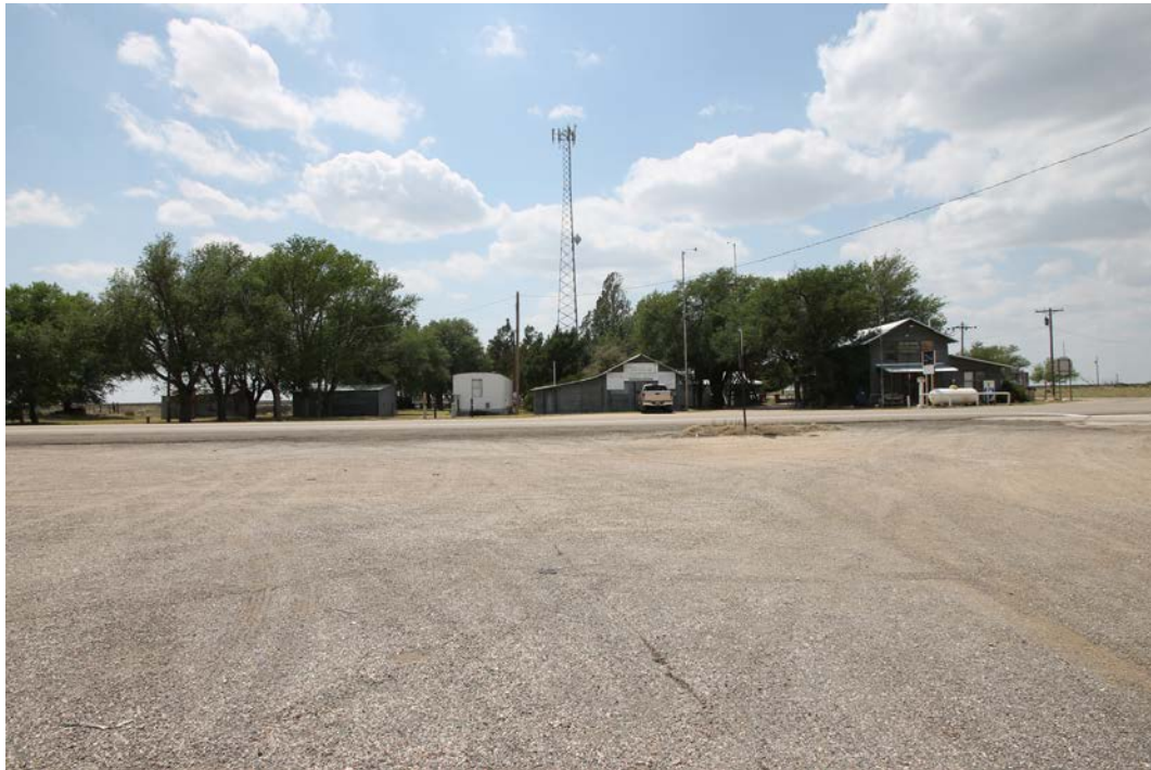
22. Davis buildings on State Highway 206, from left: garage (not in boundary), shed, mobile home, storage building and ice house, and Davis Mercantile, photographer facing west.
